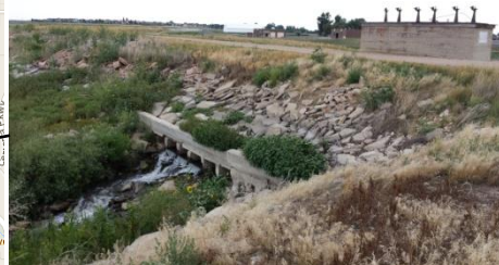
Existing Boyd Lake High-Level Outlet
