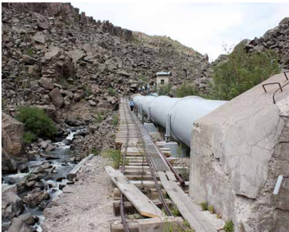
A 7-foot-diameter pipeline carries water 1.5 of the 8 miles between the Continental and Santa Maria reservoirs.
