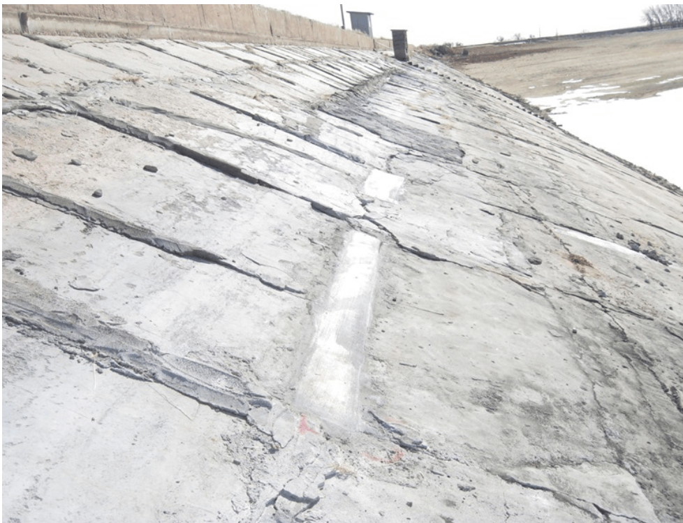
DETERIORATED & PATCHED UPSTREAM SLOPE PROTECTION
