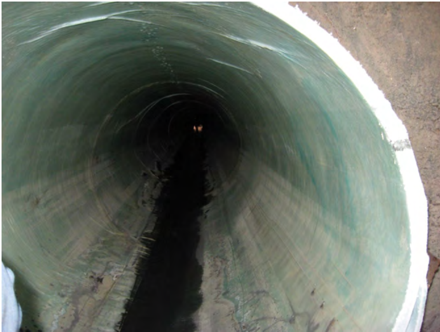
PHOTOGRAPH 9 — OUTLET CONDUIT CIPP LINING
