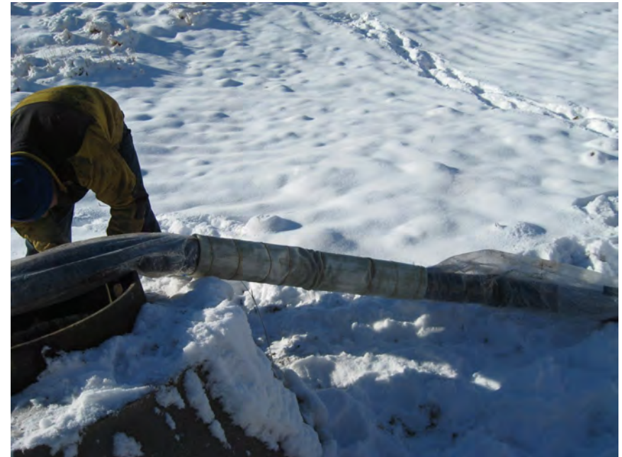
PHOTOGRAPH 12 — EXIST TOE DRAIN PATCHING
