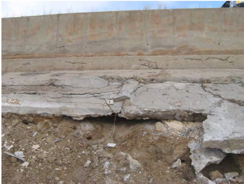
PHOTOGRAPH 3 — U.S. CONCRETE FACE DAMAGE
