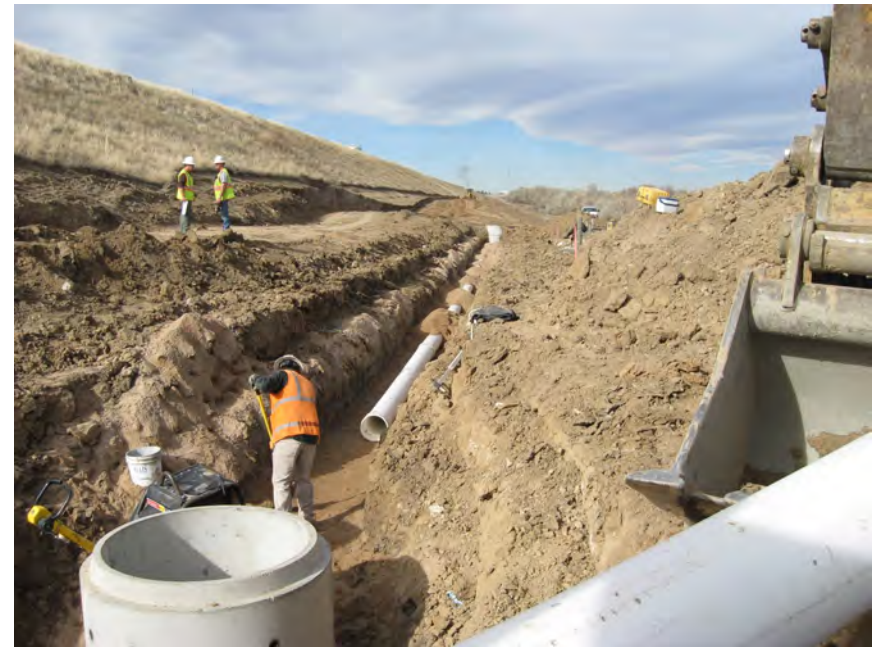
PHOTOGRAPH 10 — NEW TOE DRAIN
