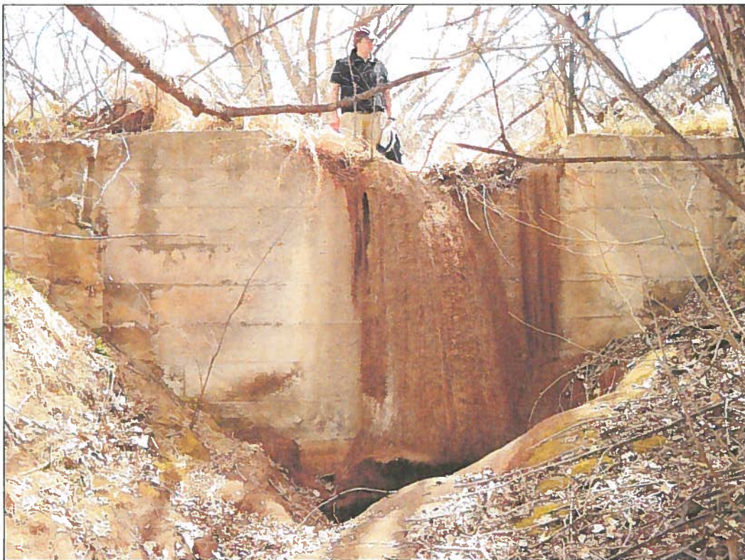
One of Three Existing Drop Structures in the Tracy Lateral
