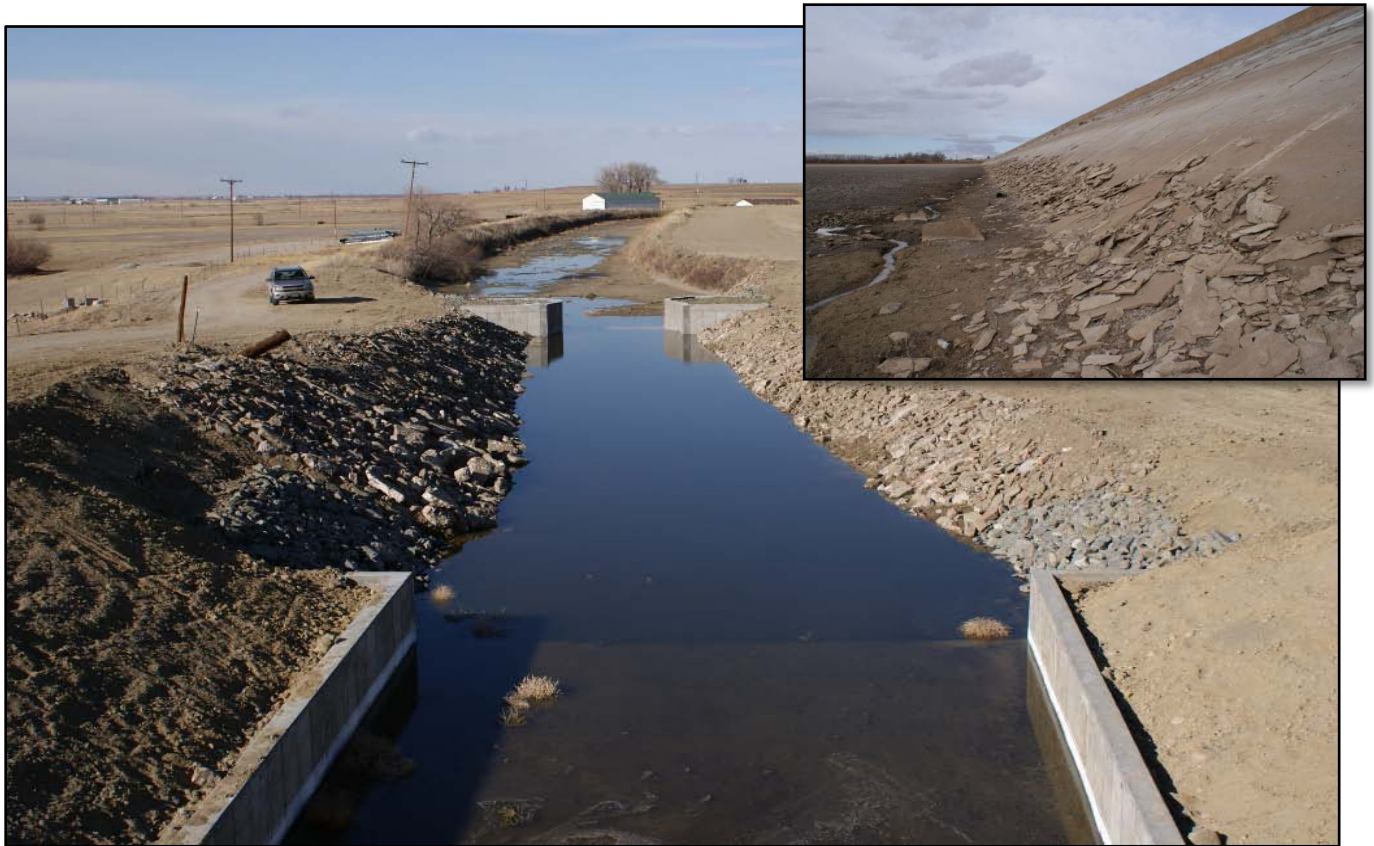
Prospect Reservoir Dam pre-project debris (inset) and the rehabilitated Horse Creek Reservoir outlet flume
