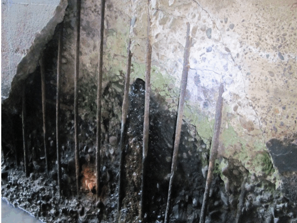
PHOTOGRAPH 5 - CONCRETE EROSION
