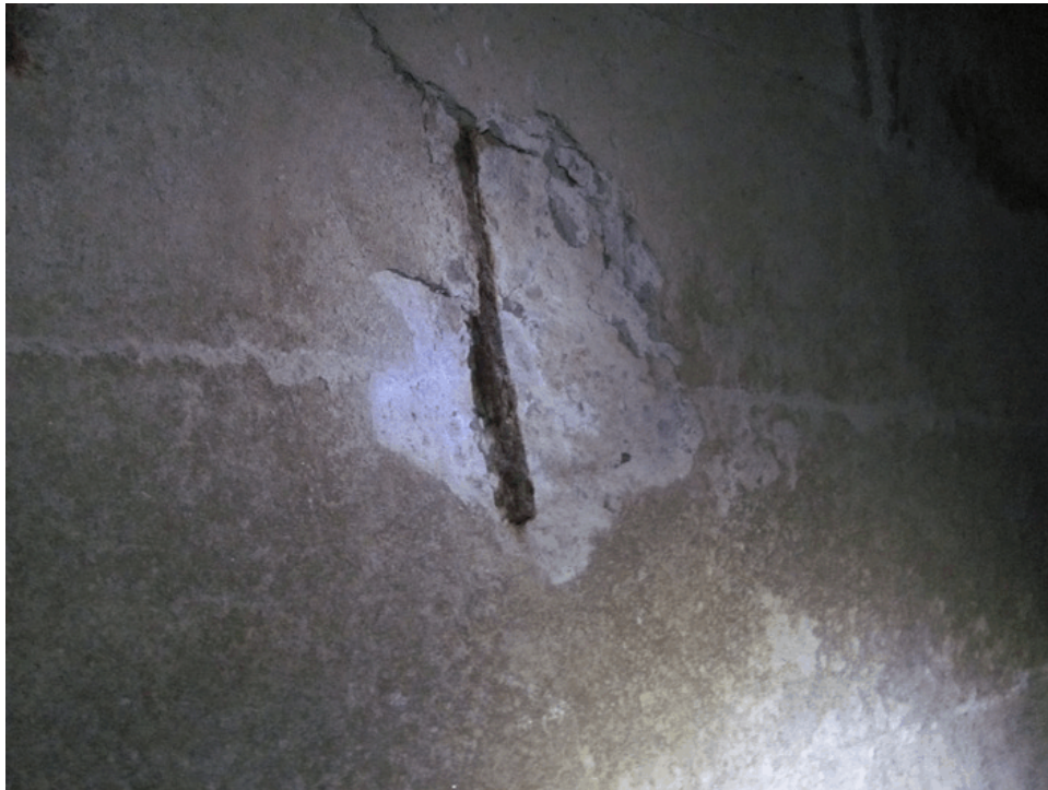
PHOTOGRAPH 9 - REINFORCING STEEL EXPOSED
