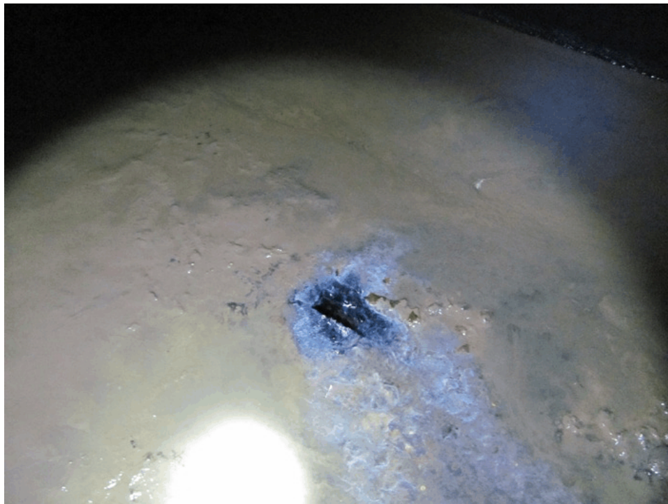
PHOTOGRAPH 10 - HOLE IN FLOOR SLAB
