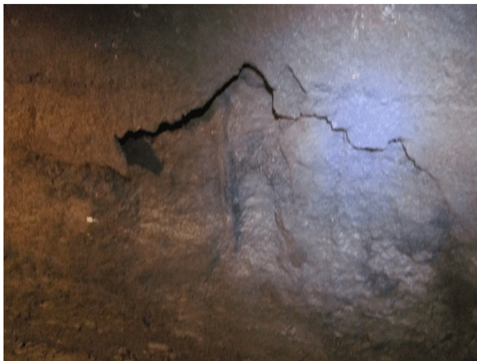
PHOTOGRAPH 8 - CONCRETE SURFACE PATCH
