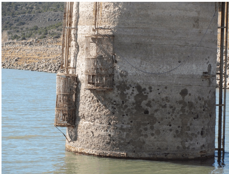
PHOTOGRAPH 2 - OUTLET TOWER DETERIORATION
