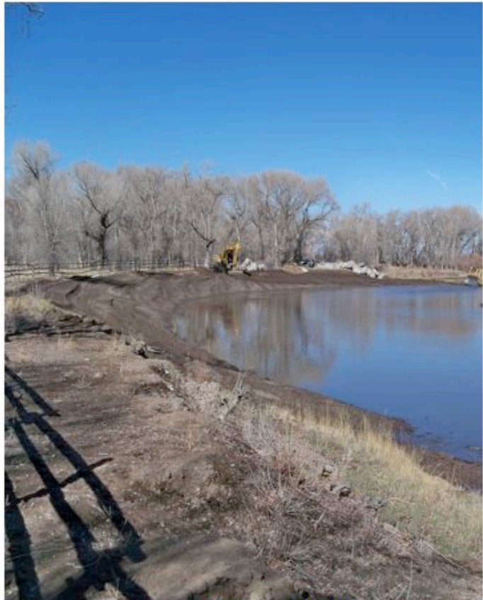
Streambank Shaping and Topsoiling.
