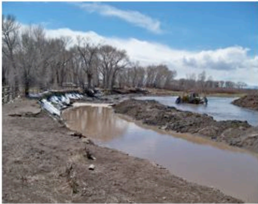
Channel and Streambank Shaping.
