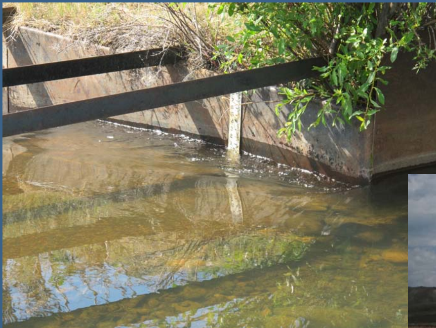
Measuring water, Parshall Flume
