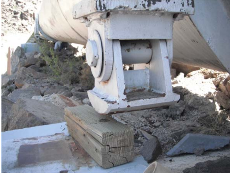
a) Rocker Supports (at S7 through S11)
