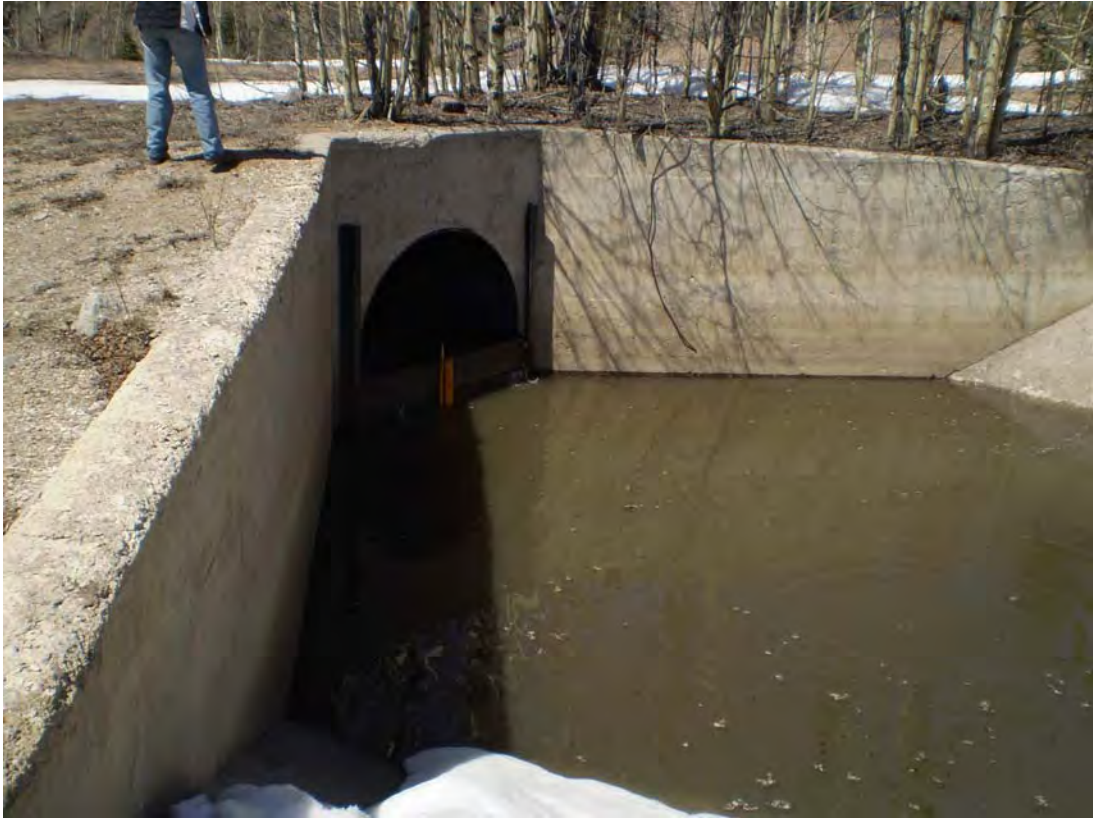
1. Siphon outlet into canal.
