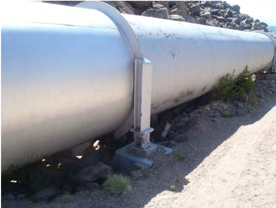
15. Looking downstream along the siphon, just upstream of the second thrust block. Seven pier support in foreground. The pier is outside of the slide area.
