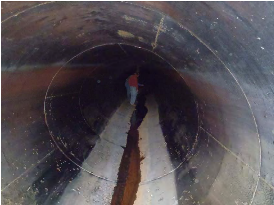
2. Inside of the discharge side of the siphon pipe.
