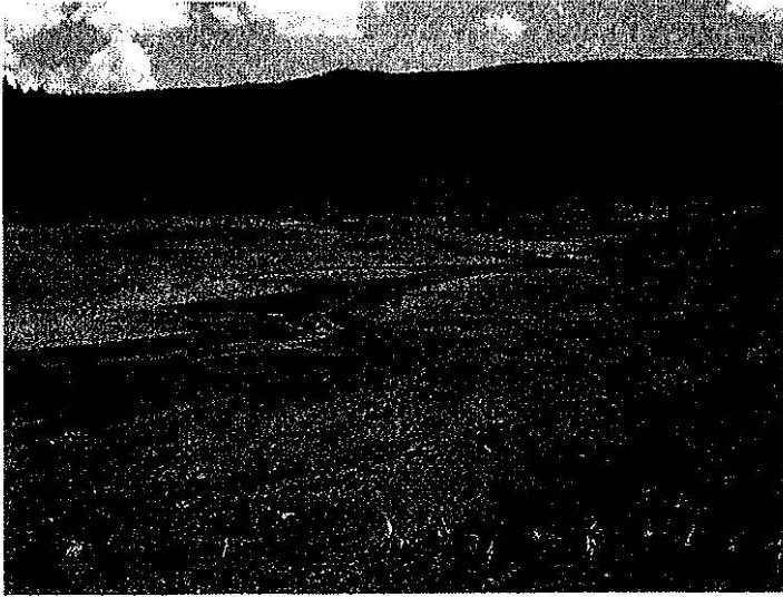
Looking at the reservoir basin from the dam crest. All fill material for an enlargement and/or rehabilitation of the dam is to come from here.
