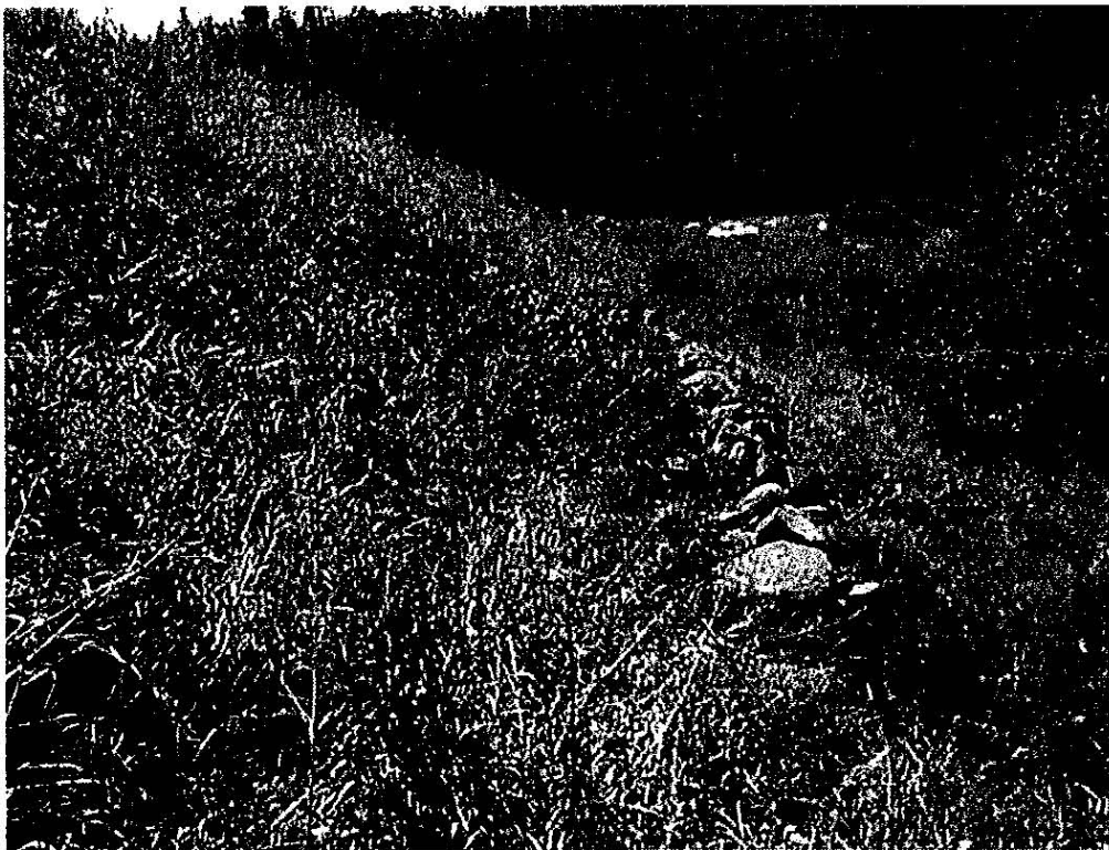
Looking at the bulging rock toe from just right of the outlet. Note depression indicating surface slide activity above the rock toe.
