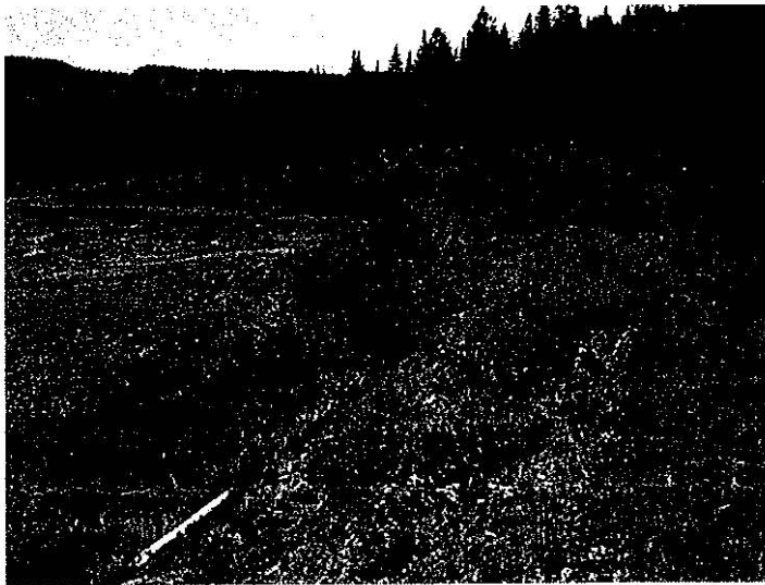
Willow growth on the northwest side of the dam that needs to be removed.
