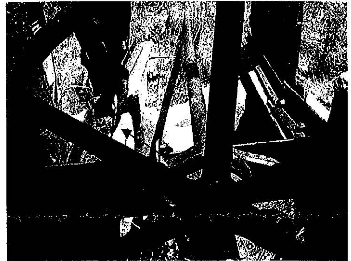
Deteriorating timbers for the outlet operator are buckling when the wheel is operated. Note gap between steel structure and timbers that was created by this buckling.
