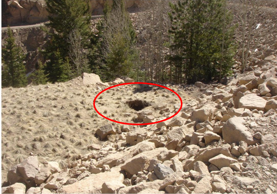
Photograph No. 8 View from crest dike looking downstream at the 2010 sinkhole.
