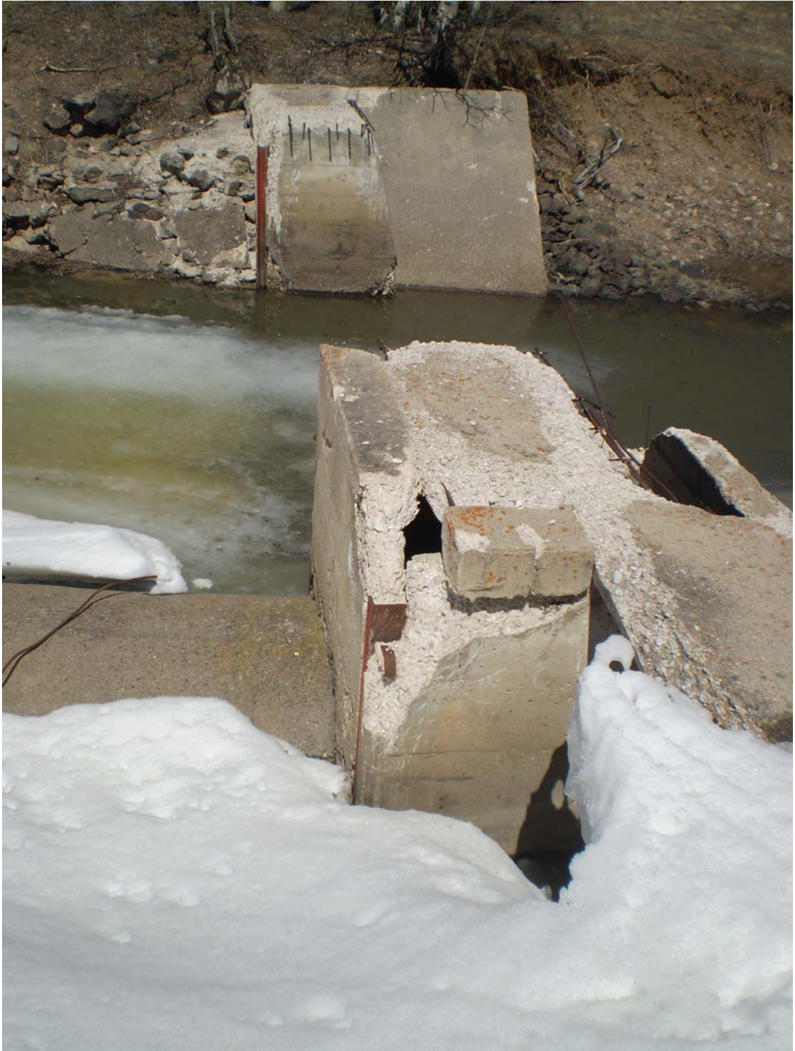
5. Control structure just downstream of the siphon outlet structure.
