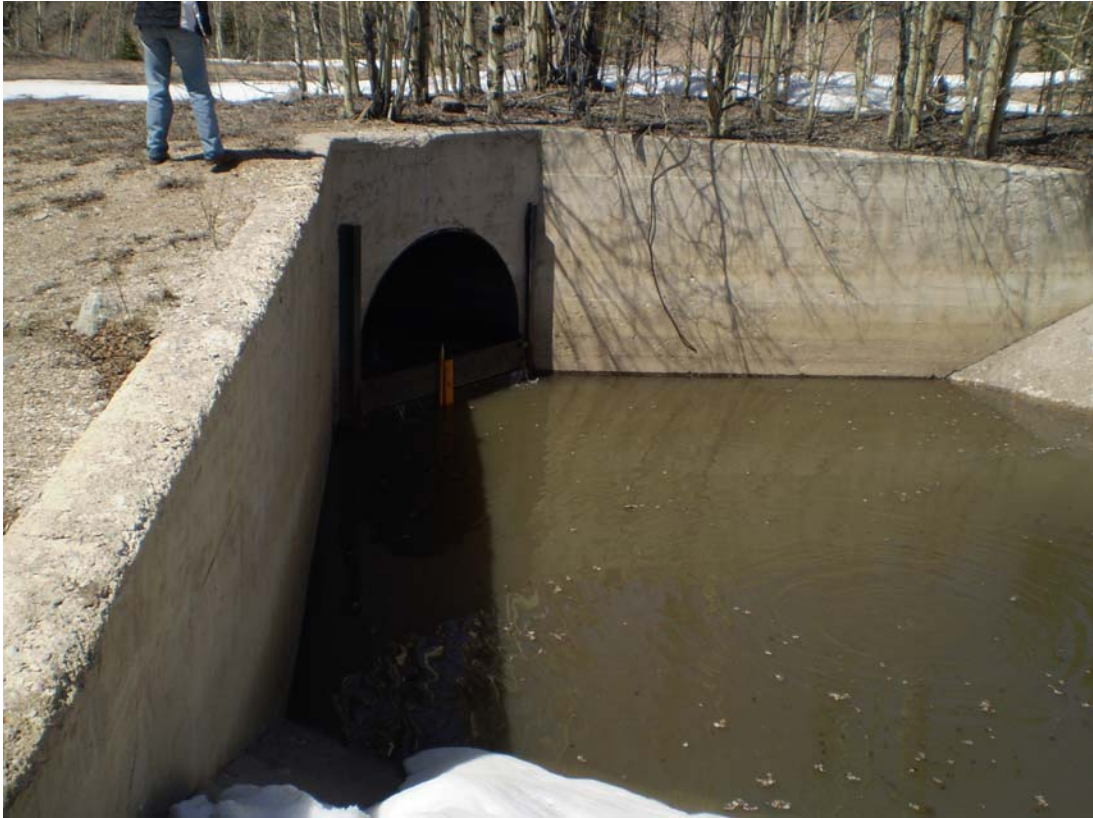
1. Siphon outlet into canal.
