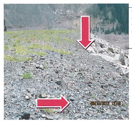
This picture shows the "sloughing" of the edges and the rounding effect of the rock settling, this exposes the small rock to wind erosion that could ultimately expose the core.
