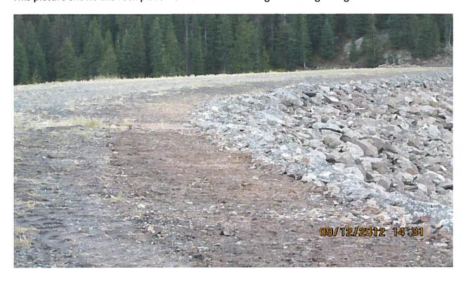
This is after the final gravel and grading. Notice the orange outline, this is a survey settlement point for the dam.
