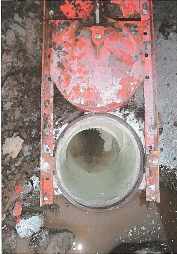
Figure 9 Water-tight seal at the slide gate.
