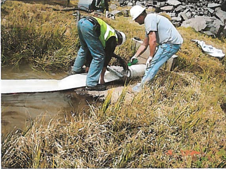
Figure 4 Checking the alignment of the liner feeding through the rollers.
