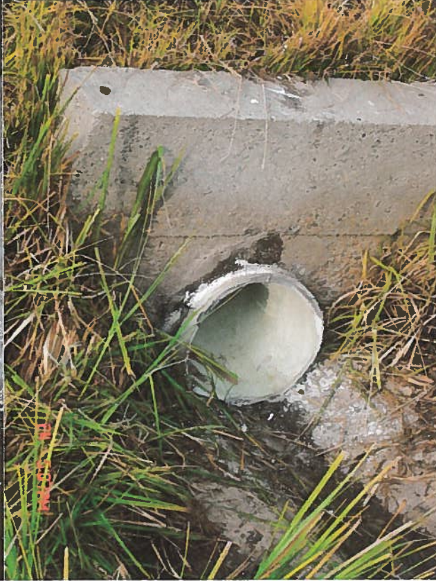
Figure 10 Finished CIPP at the outlet of the reservoir.
