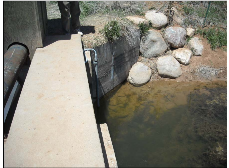
Photo 14: Pastorius Reservoir outlet with staff gauge.
