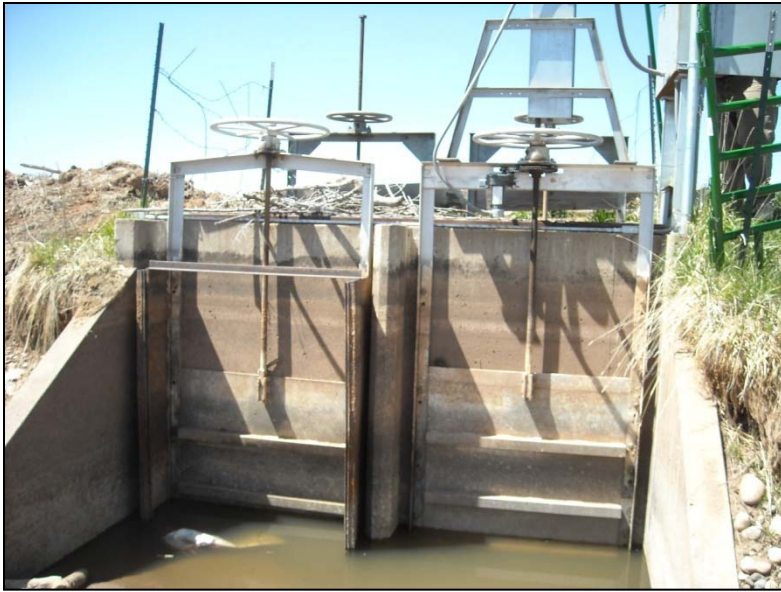
Photo 1: Florida Farmers Ditch West turnout – actuated slide gates.
