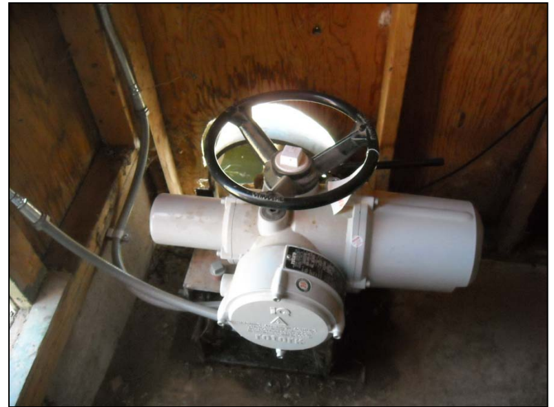
Photo 16: Pastorius Reservoir – gate actuator (by Rotork).
