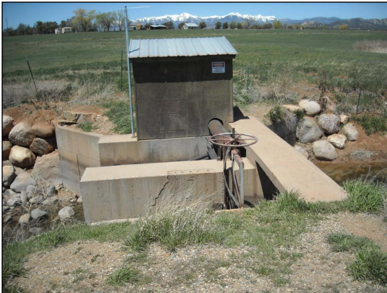
Photo 19: Gate and control house at Pastorius Reservoir outlet.
