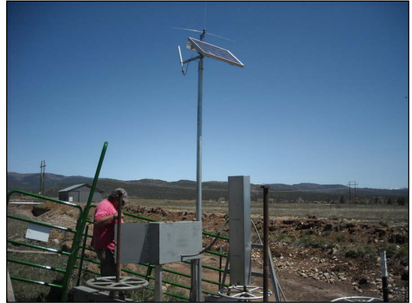
Photo 6: Florida Farmers Ditch West – panel, actuator, solar panel and antenna.
