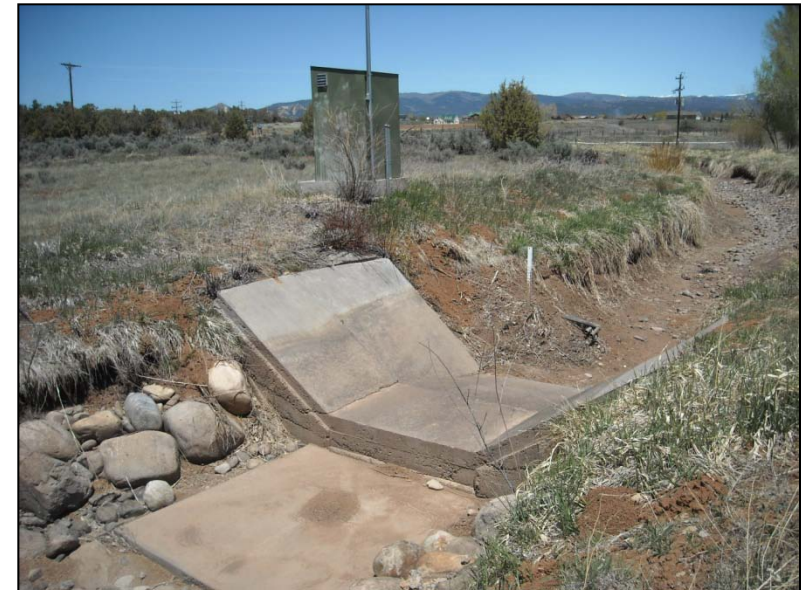
Photo 20: Influent to Pastorius Reservoir - stilling well house with level measurement.
