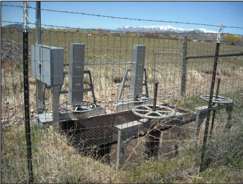
Photo 11: Pine Ditch turnout – actuated gates with control panel.
