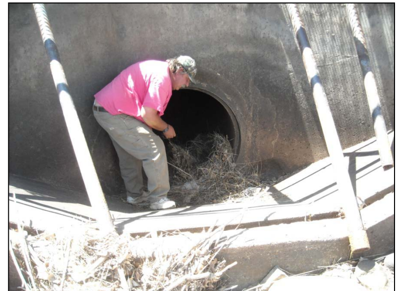
Photo 12 Mankiller inlet. 40" Ø pipe, 120' long 20' drop.
