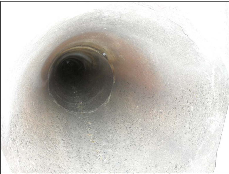
Photo 3 Drop #1: 36-inch Ø RCP penstock – 80' long, 20 foot fall.
