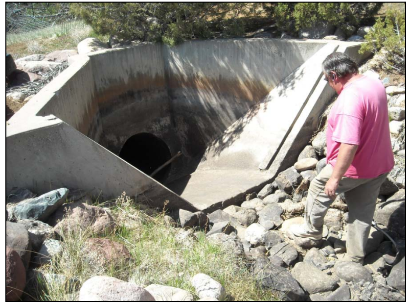
Photo 2 Drop #1: Penstock inlet.
