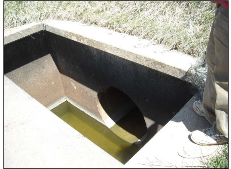
Photo 10 Drop #4. Outfall of penstock downstream from confluence.
