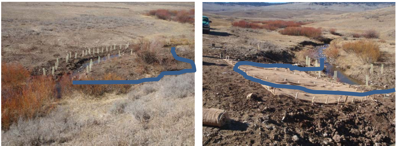
Figure 1 – Site 1 (left) with new channel construction and Site 5 (right) with hardened streambank and floodplain. The blue line represents the old (i.e., pre-restoration) channel.
