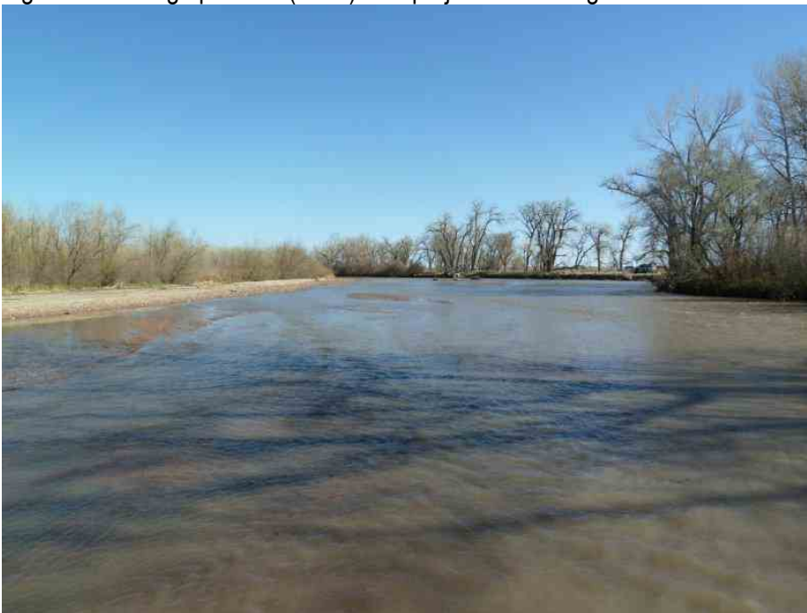
Figure 4: Looking upstream (north) with project area on right. Creek is too wide and will be reduced to 160ft width.
