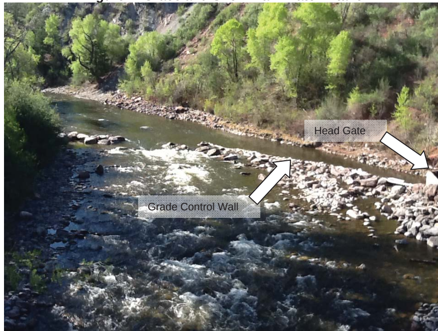
Figure 1. Grace and Shehi Raw Water Intake
