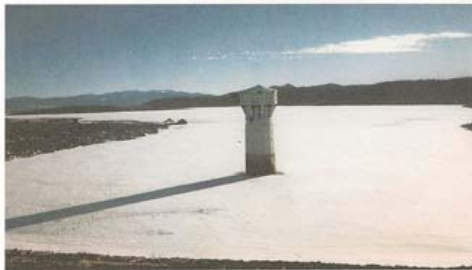
Sanchez Reservoir Gate Tower and Outlet Repairs involved the removal of the original (1917) manually operated gates with new gates and hydraulic operators.
