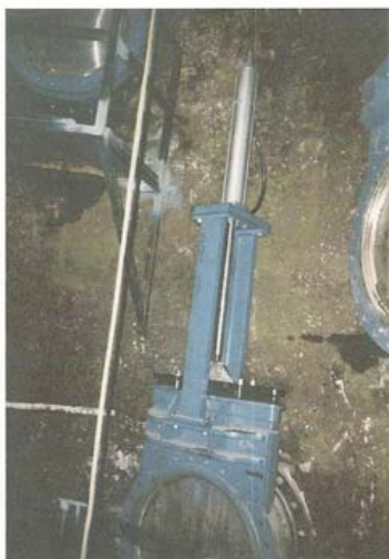
Sanchez Reservoir Gate Tower and Outlet Repairs involved the removal of the original (1917) manually operated gates with new gates and hydraulic operators.
