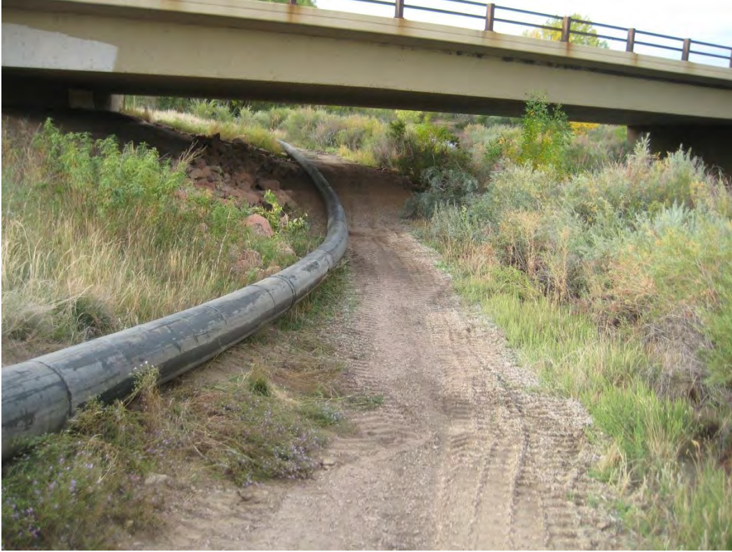
Figure 4. Typical Installation of 18-inch Diameter Bypass Piping at Road Crossing
