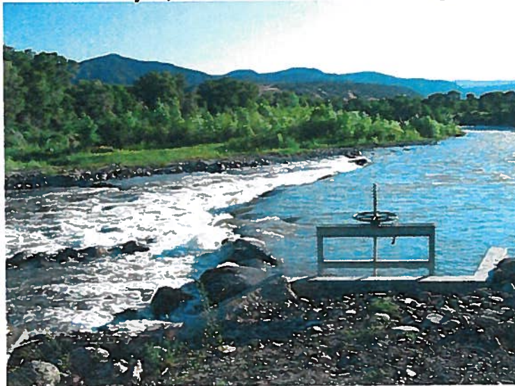
Figure 2. Successfully Rehabilitated Linear Grade Control Wall (NFRIA-WSERC Conservation Center, North Fork of the Gunnison River Restoration Project, www.theconservationcenter.org )
