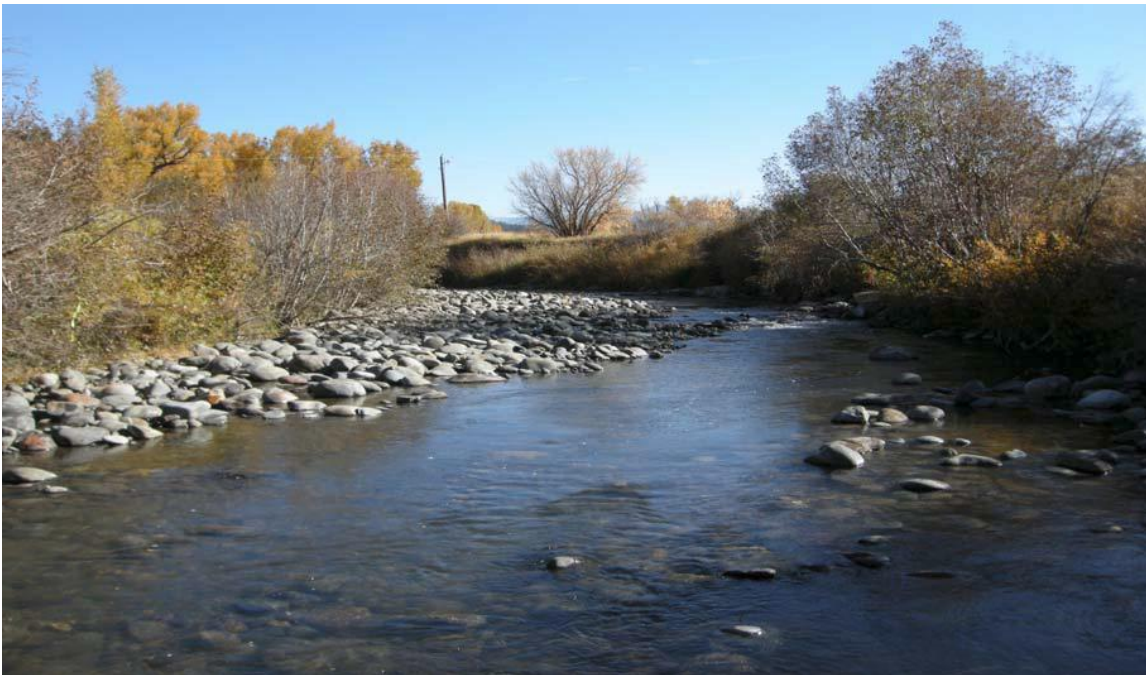
Typical Restored Section. Photo of newly constructed point bar with dense bank vegetation. Note the rock structure and deeper water river-left, creating good fish holding potential beneath the overhanging riparian vegetation.
