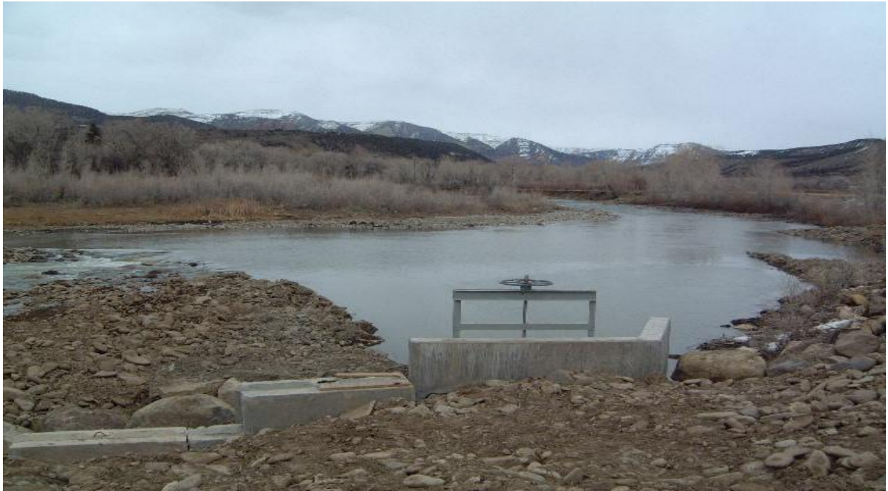
Paonia headgate at project completion.
