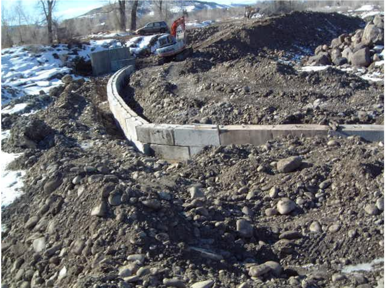
Diversion footing under construction.
