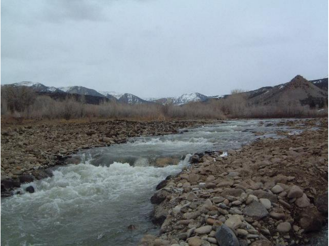
Completed plunge pools below diversion.
