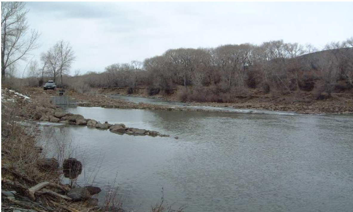
Rock vein protecting bank above Paonia headgate.
