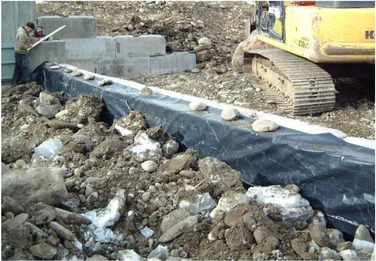
Sealing diversion footing.
