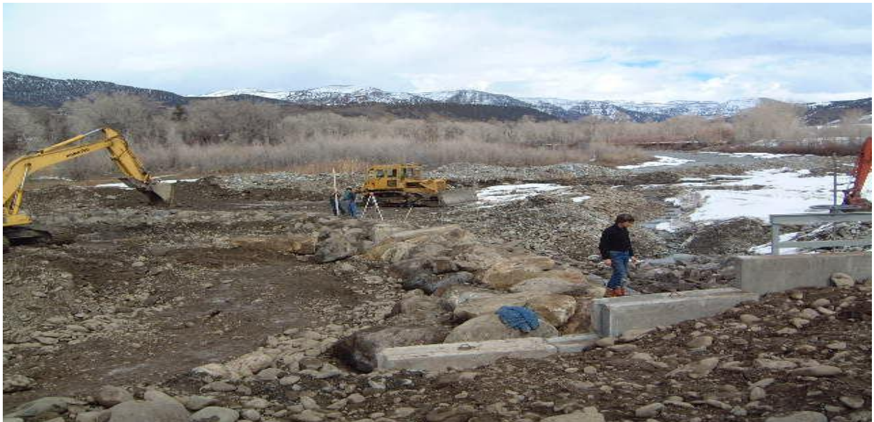
Placing boulders in diversion structure.
