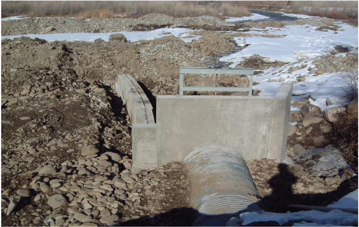
Paonia headgate during construction.
