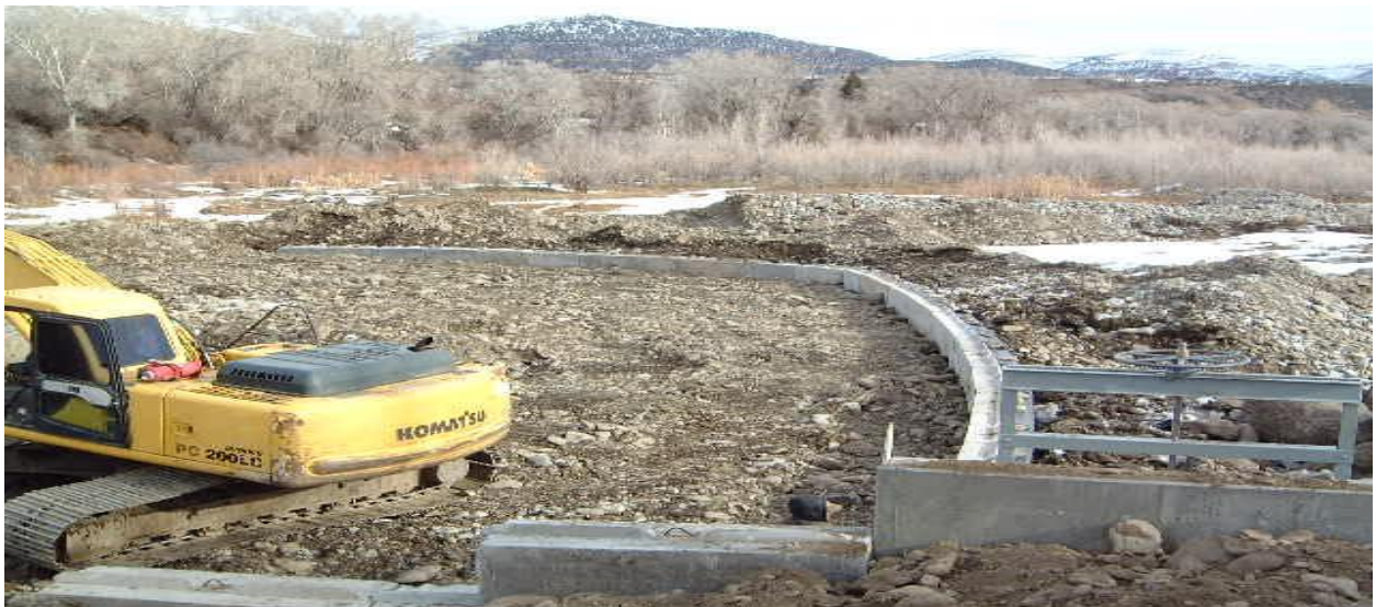
Construction of diversion footing.
