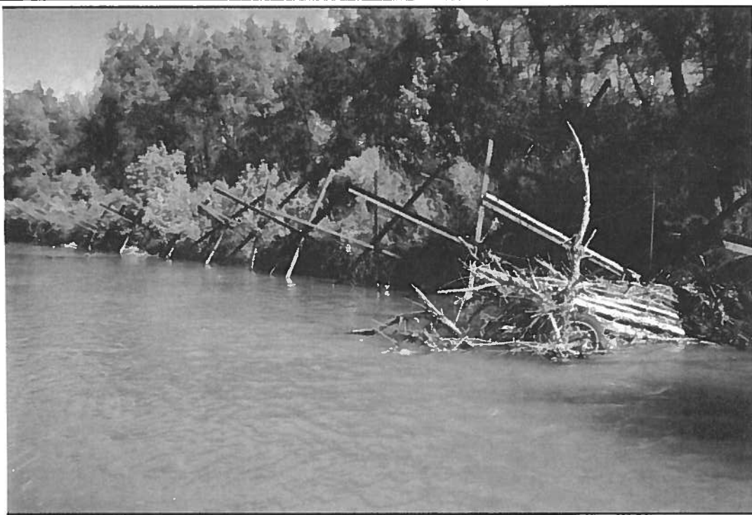
Failed Jetty-Jack bank stabilization structures in Reach 3 of the Purgatoire River.
