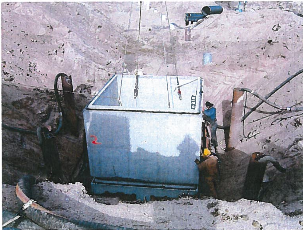
WET WELL MIDDLE SECTION PLACEMENT
