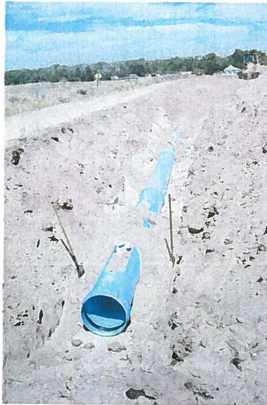
24" PIPE INSTALLATION APPROX. STA 10 + 00
