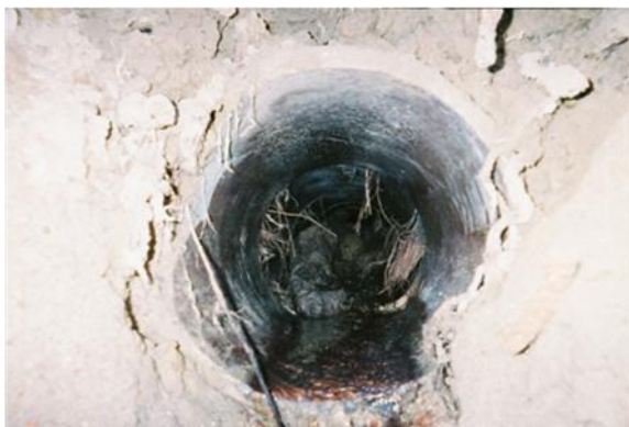
Obstructions in Tile Line Before Cleaning
