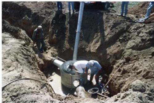
Tile Line Penetration - Installing and then cleaning out a manhole in order to clean an otherwise inaccessible plugged tile line – (1) Carefully excavating tile line to install manhole at bend; (2) Installing manhole, connecting pipe, and use of vacuum to assist installation; (3) Completing installation; (4) vacuuming silt out of manhole after the plugged tile line has been cleaned.
