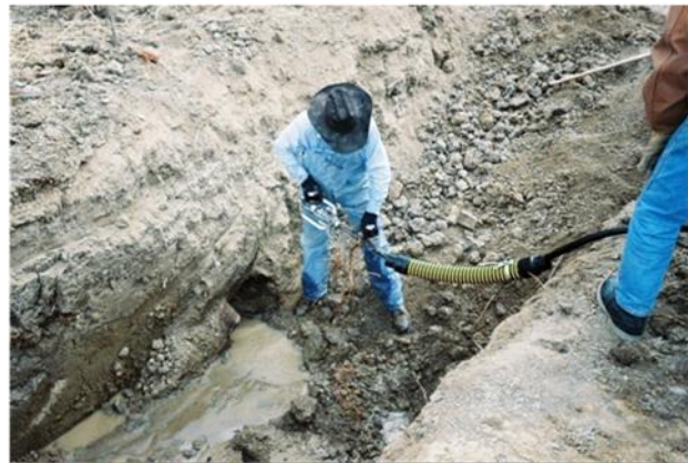
Cleaning roots off nozzle
