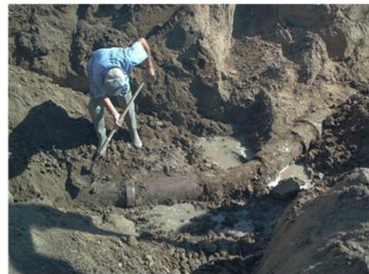
Exposing a Tile Line Before Installing a Manhole
