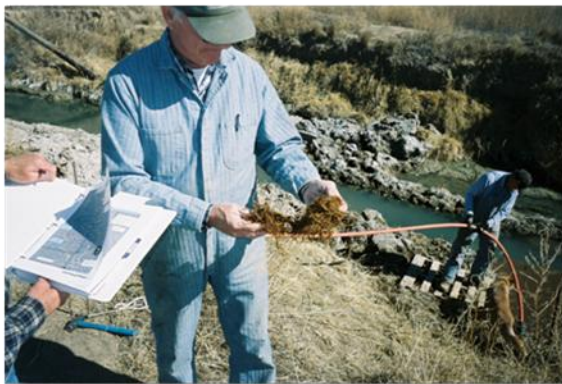
(1) Rural subdivision encroachment onto open drain; (2) Bell tile joint; (3) Cleaning alfalfa roots out of a tile line; (4) Typical sink hole in middle of field.
