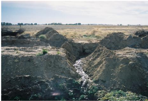
Typical Tile Line Outlet with Effluent Flowing into Open Drain (forefront)
