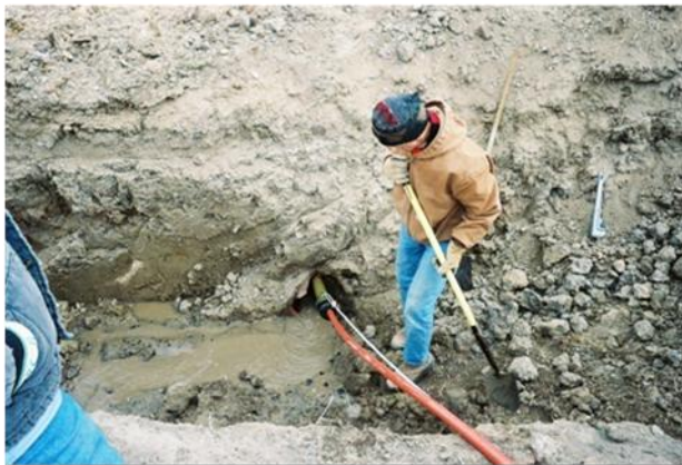
Working (moving in and out of) tile line
