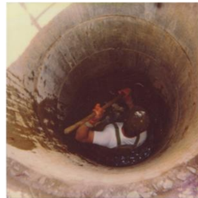
South Columbia Basin Irrigation District (three man drainage crew) – (1) Dan Morasch, Technician (retired); (2) total field crew for 1200 miles of tile lines and 3000 manholes; (3) Cleaning a root ball out of a manhole; (4) Cleaning out a manhole. Their maintenance program is discussed later in the report.
