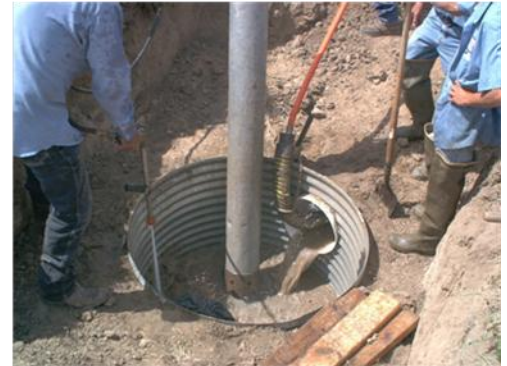
Tile Line Penetration - Installing and then cleaning out a manhole in order to clean an otherwise inaccessible plugged tile line – (1) Carefully excavating tile line to install manhole at bend; (2) Installing manhole, connecting pipe, and use of vacuum to assist installation; (3) Completing installation; (4) vacuuming silt out of manhole after the plugged tile line has been cleaned.
