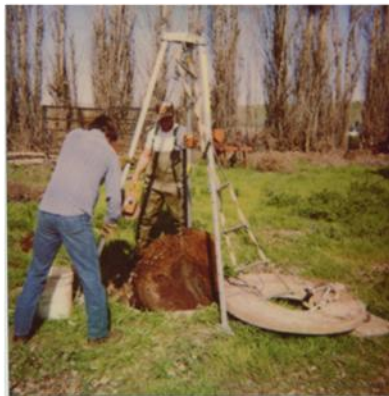
South Columbia Basin Irrigation District (three man drainage crew) – (1) Dan Morasch, Technician (retired); (2) total field crew for 1200 miles of tile lines and 3000 manholes; (3) Cleaning a root ball out of a manhole; (4) Cleaning out a manhole. Their maintenance program is discussed later in the report.
