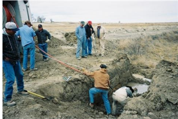
Running nozzle and hose into tile line
