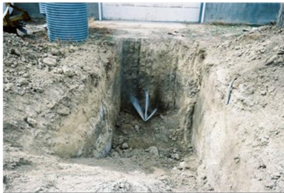
Demonstration tile line cleaning on George Reyher farm – (1) Inserting nozzle and hose into tile line; (2) Waiting for the “wart hog” (high pressure nozzle) to pass through the plugged 800 foot long 8” diameter line; (3) Jet nozzle exiting tile line where a new 6’ diameter galvanized pipe manhole (above left) is planned; (4) Aerial view of the cleaned tile line on Reyher farm.
