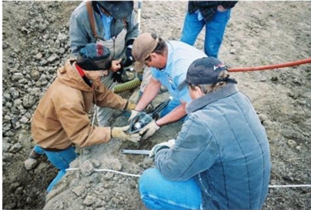
Attaching high pressure nozzle to 1" water hose.
