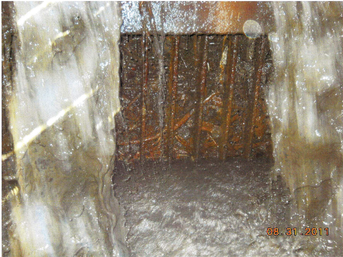
View of silted in lower level intake and trashrack looking upstream.
