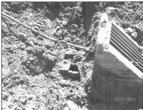
The photograph on the left shows the excavation of the wooden conduit behind the intake structure. The photograph on the right shows the interior of the wooden conduit within the impacted area.
