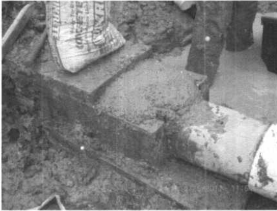
The photographs on the left and right shows the PVC piping grouted into place.
