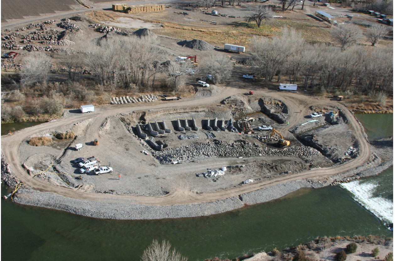
Construction progress November 22, 2011
