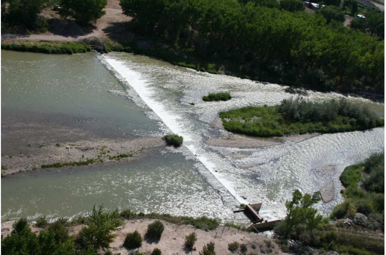
Arial View prior to construction
