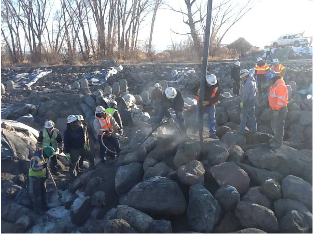
Grouting structures in boat passage.
