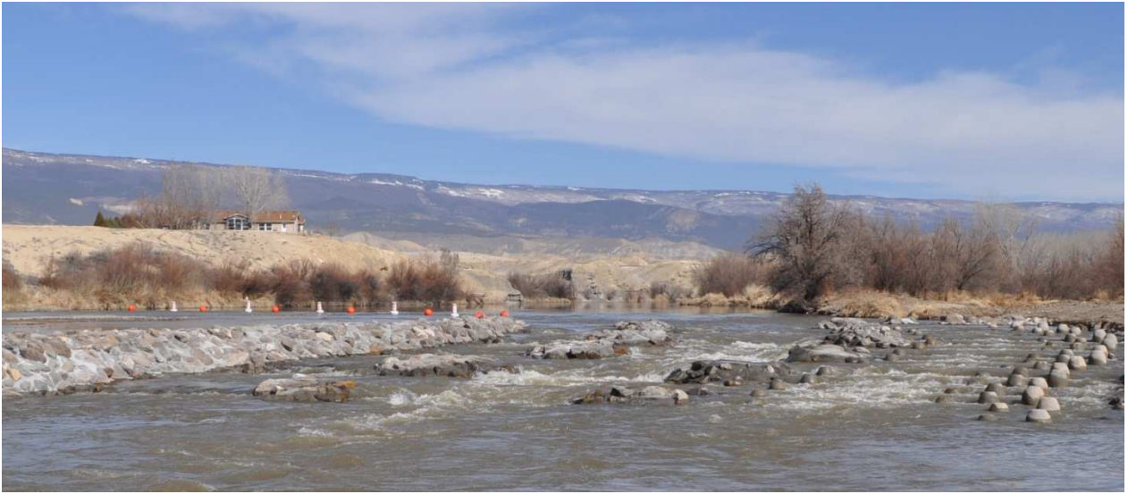
Figure 2 – Hartland Dam Fish and Boat Passage
