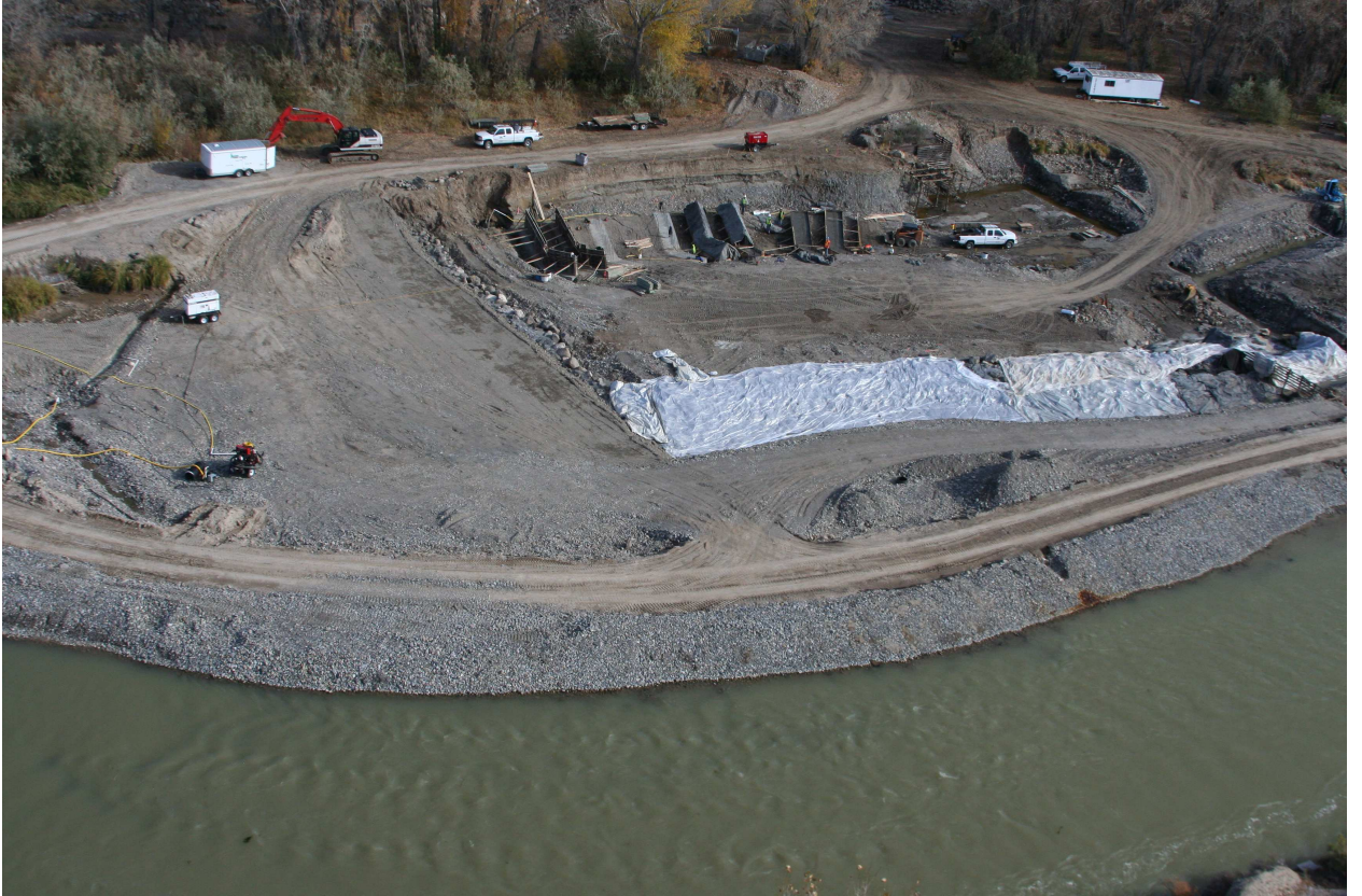
Construction progress October 13, 2011
