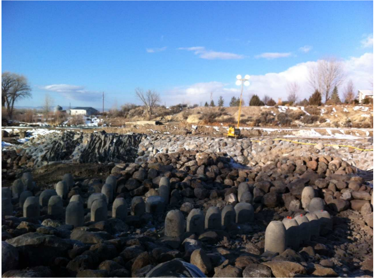
Standing on river bank looking across project
