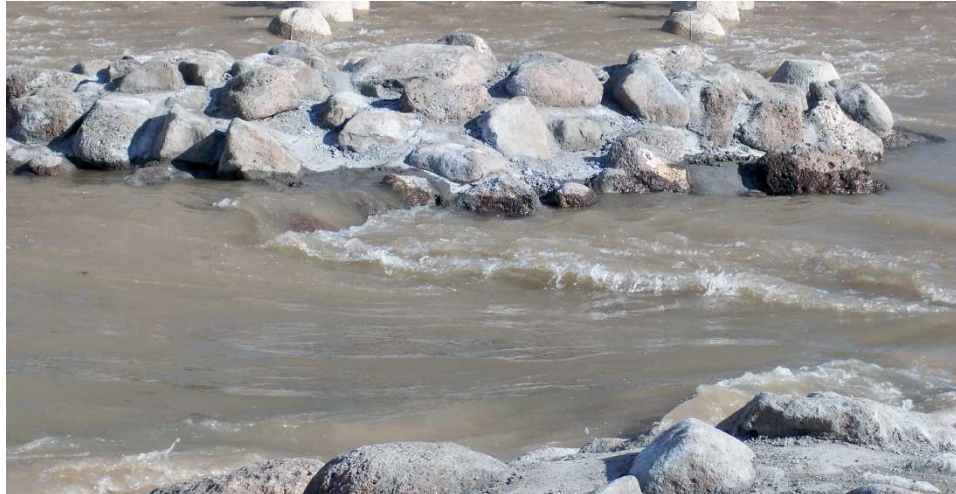
Figure 6 – Grouted Boulders
