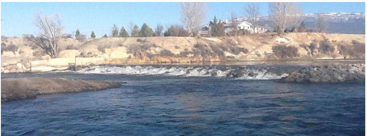
Dam modifications completed.
