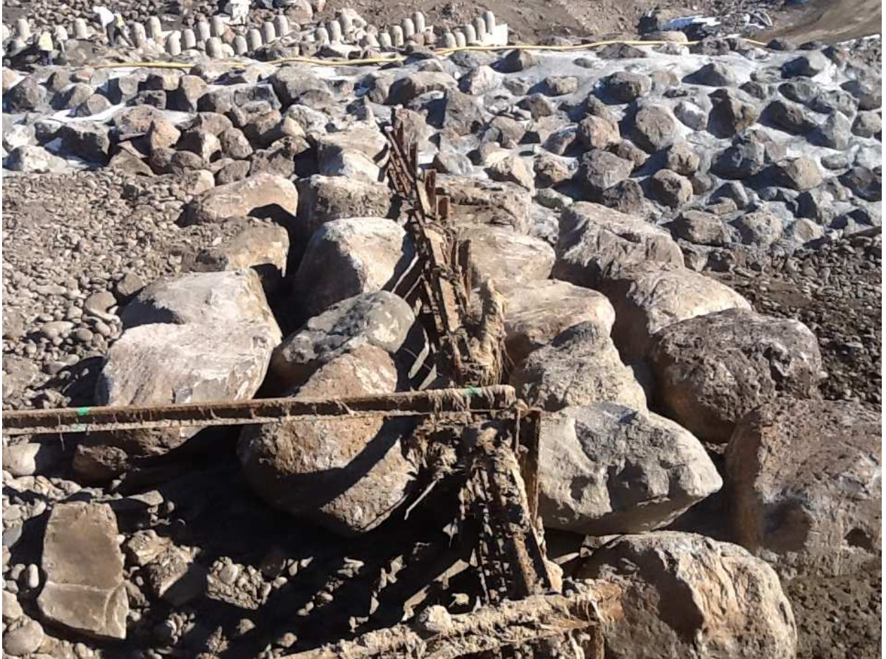
Dam modifications to remaining existing dam
