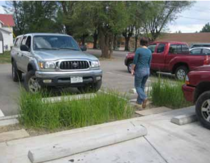
Right: Stormwater from a parking lot is filtered through native vegetation at Ignacio Public Library. The design provides for water quality as well as providing stormwater that sustains the vegetation.
