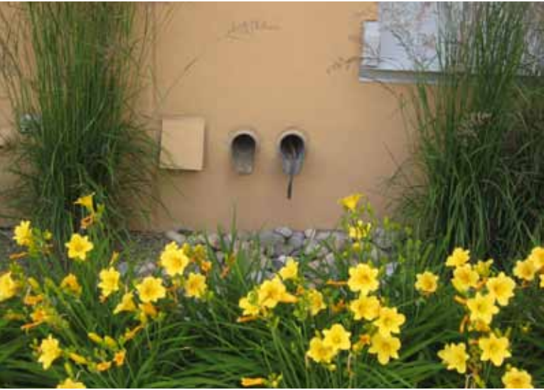
Left: Roof run-off is directed off the roof and into native vegetation.
