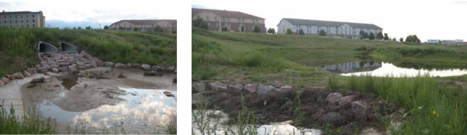
The image to the left is a hardened forebay that collects sediment and the image to the right is a series of ponds that filters containments. Both images are from the Highpoint development near Denver International Airport.
