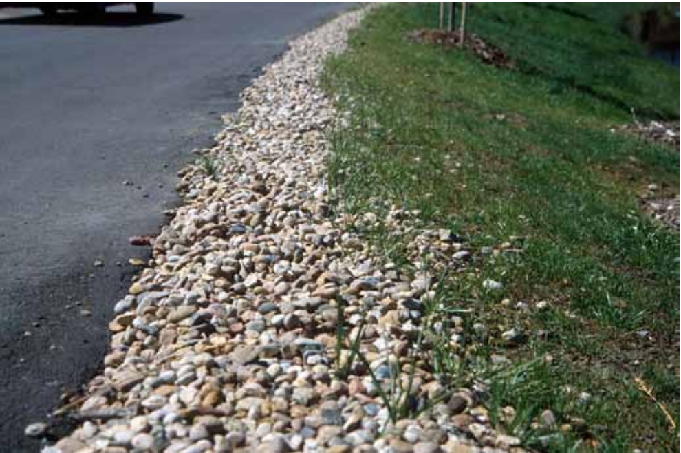
A gravel filter strip that collects sediment from the roadway.
