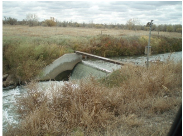
Drop structure downstream of ditch head gate
