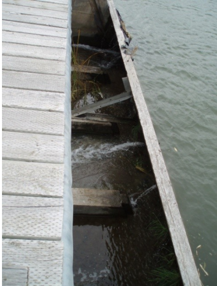
Looking down at wooden stop logs
