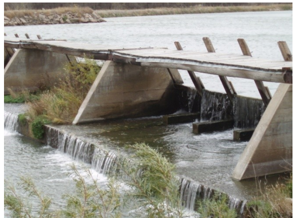
Concrete piers and wooden stop logs
