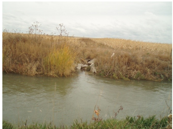
Incoming field drain with erosion
