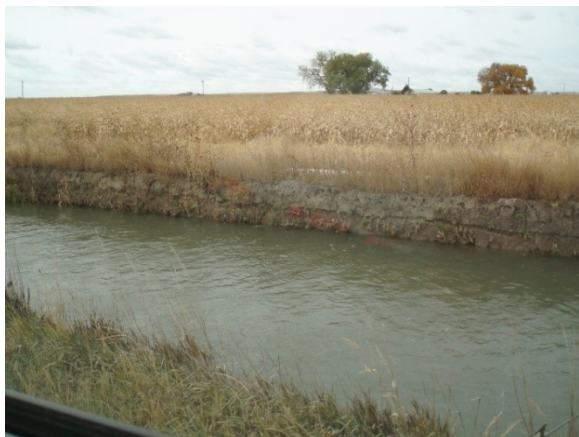
Near vertical wall & seepage along north embankment
