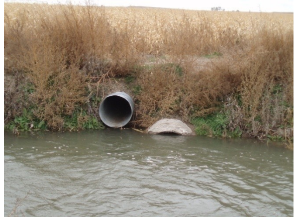
Field drains in the north embankment
