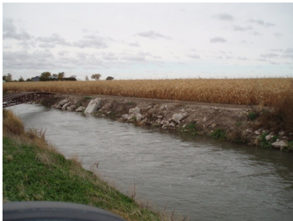
Erosion along the north embankment
