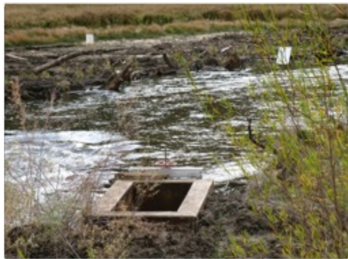
Above and left: forming and pouring the new diversion. Finished diversion, fed by a double cross weir (below), which is designed to be able to deliver water in all flow regimes.
