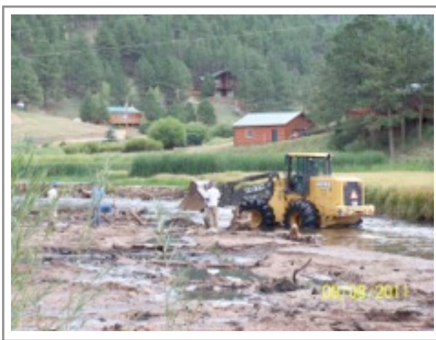
Narrowing the stream back up just above the dam site, where it had over-widened over decades and threatened the road. On left, filling, on right replanted with sedge and willows.
