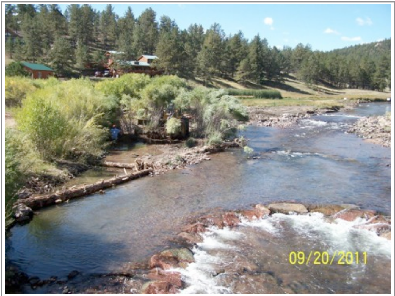
Looking upstream, where the dam once blocked the river. The cross-weir in the foreground guides the thalweg into the middle of the area as the water flows under a bridge.
