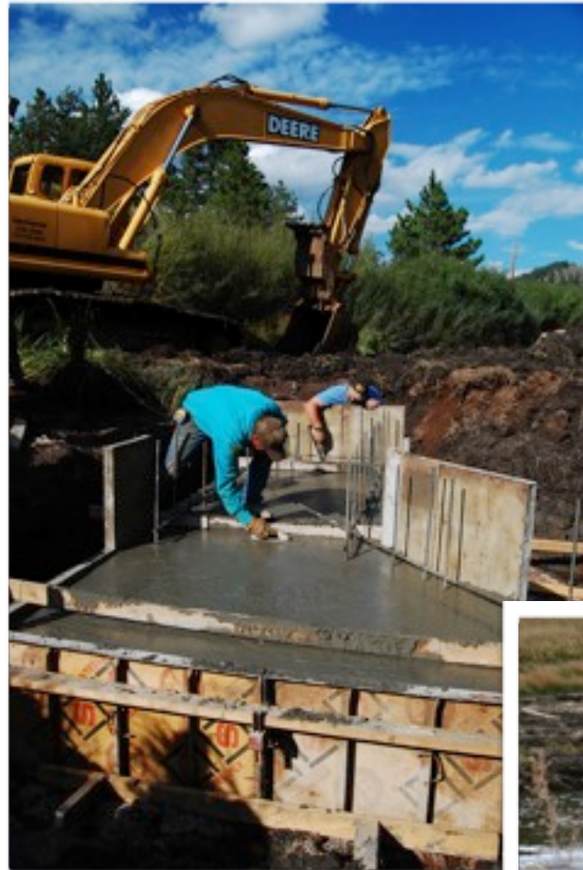
Above and left: forming and pouring the new diversion. Finished diversion, fed by a double cross weir (below), which is designed to be able to deliver water in all flow regimes.
