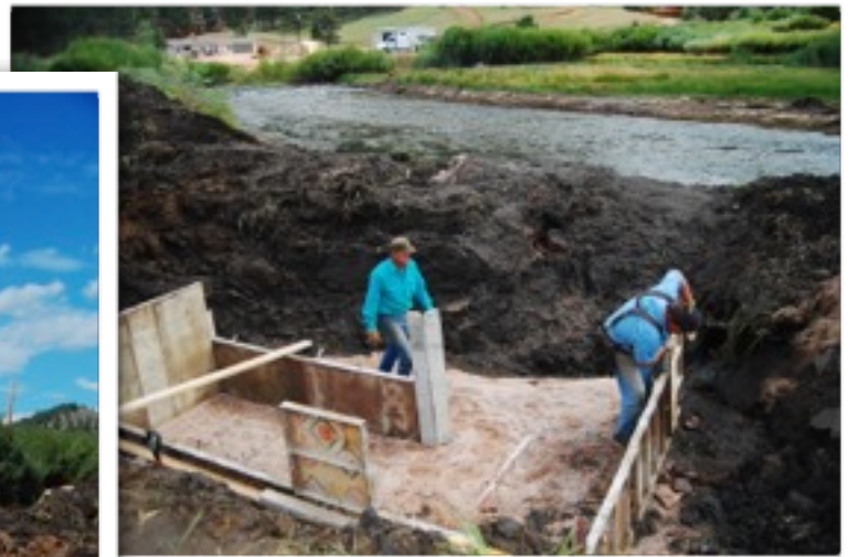
Above and left: forming and pouring the new diversion. Finished diversion, fed by a double cross weir (below), which is designed to be able to deliver water in all flow regimes.
