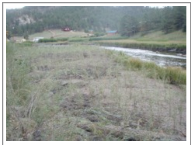
Narrowing the stream back up just above the dam site, where it had over-widened over decades and threatened the road. On left, filling, on right replanted with sedge and willows.
