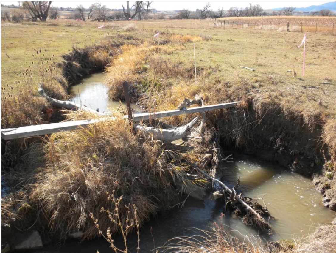
This photo shows the erosion of Rock Creek stream banks, prior to restoration work.
