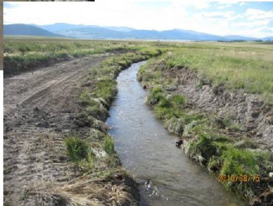
Figure 9 Before-after of bench/floodplain treatment on the upper segment just after construction in August, 2010
