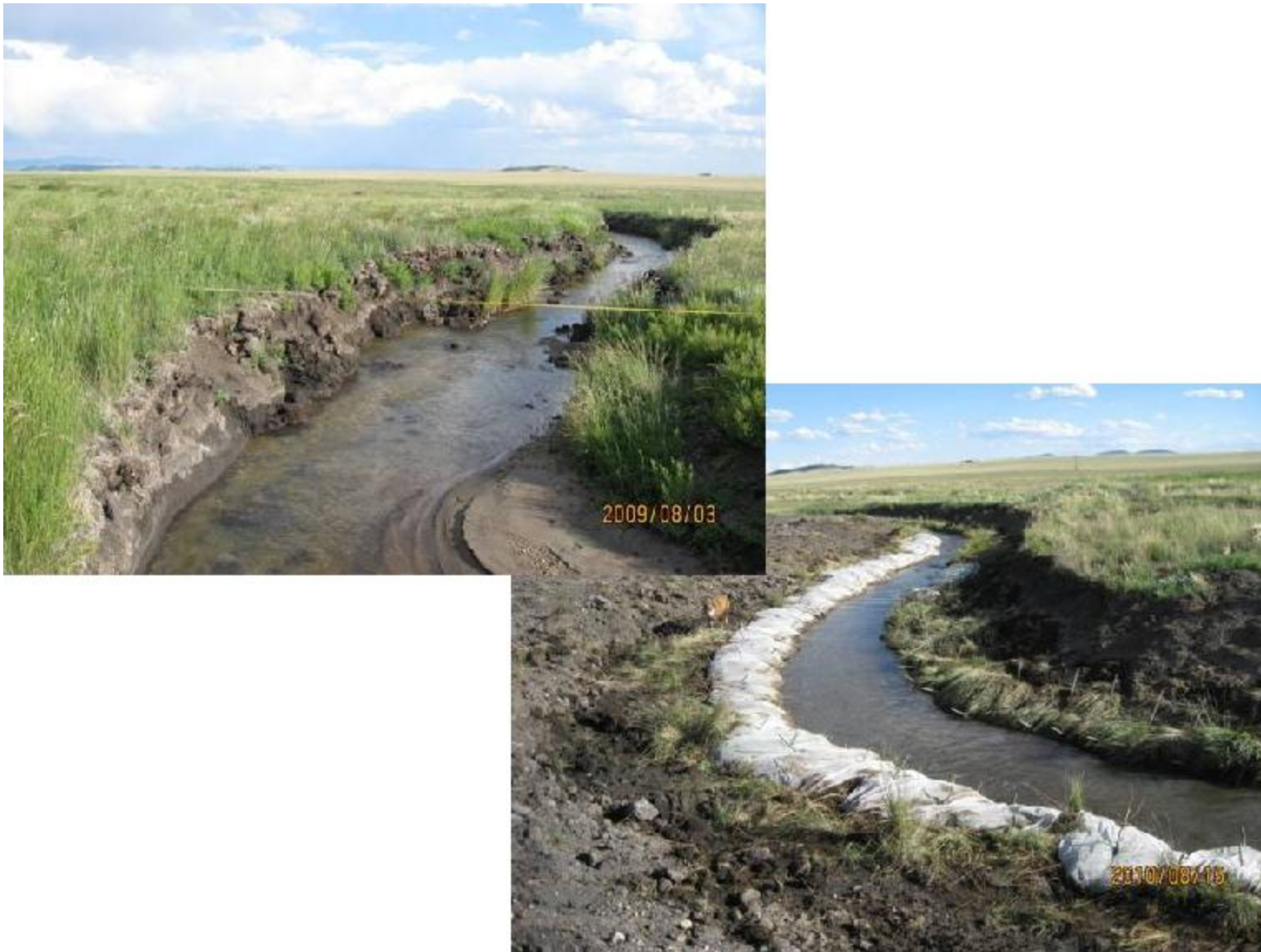
Figure 11 Before-after of bench/floodplain treatment on the upper segment just after construction in August, 2010
