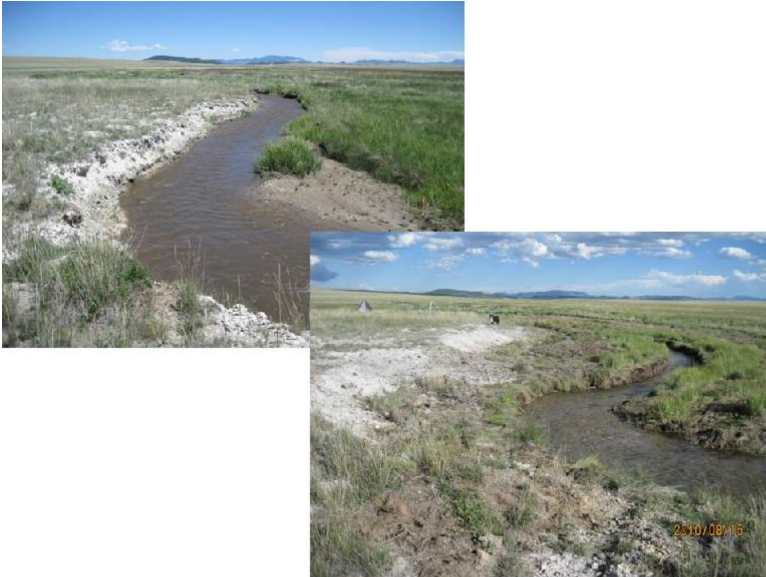
Figure 16 Before-after of channel realignment treatment on the upper segment just after construction in August 2010.
