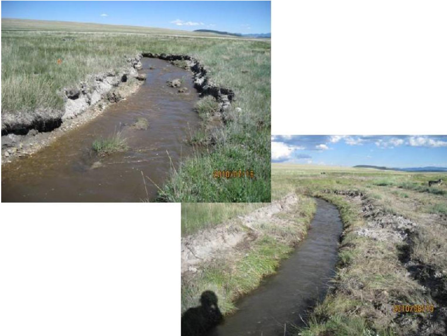
Figure 10 Before-after of bench/floodplain treatment on the upper segment just after construction in August, 2010
