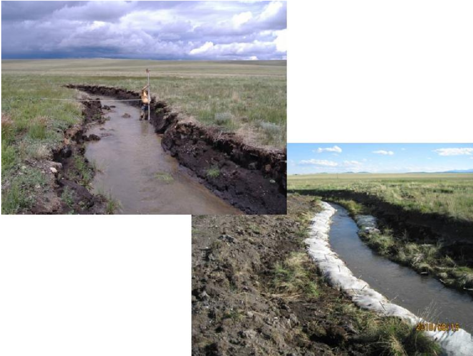
Figure 12 Before-after of bench/floodplain treatment on the upper segment just after construction in August, 2010
