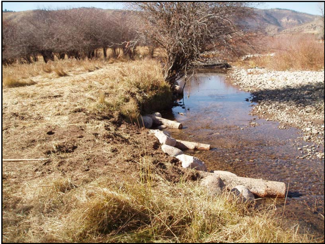
Point 1V13L: 10-30-08 Pre-planting, looking downstream at recently-installed log-rock deflectors.
