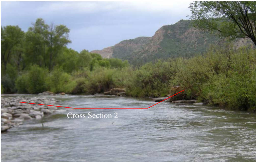
Cross Section #2 After construction looking downstream. Newly constructed point bar river left and rock habitat clusters river right.
