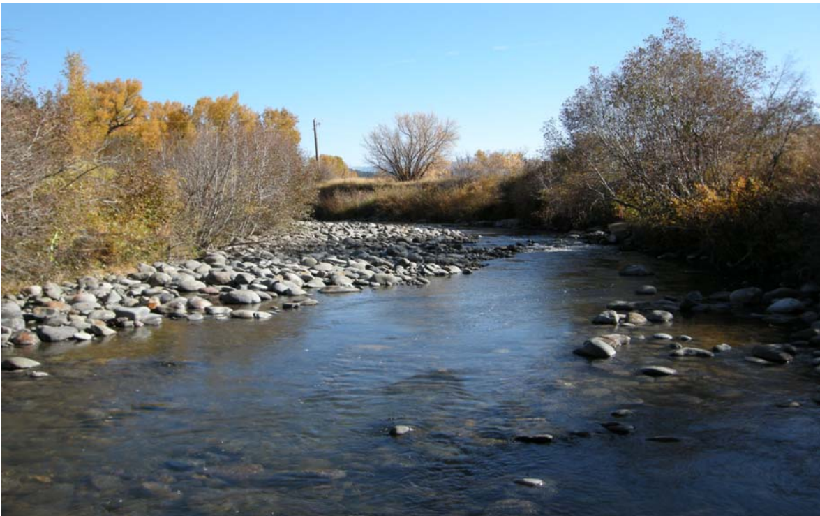
Typical Restored Section. Photo of newly constructed point bar with dense bank vegetation. Note the rock structure and deeper water river-left, creating good fish holding potential beneath the overhanging riparian vegetation.
