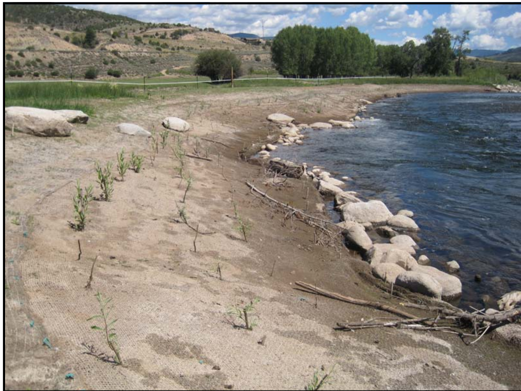
Point 2V3R: 8-15-11 Treatment area 2-6 after bank layback, ditch abandonment, willow wattle installation, and cobble toe reinforcement.
