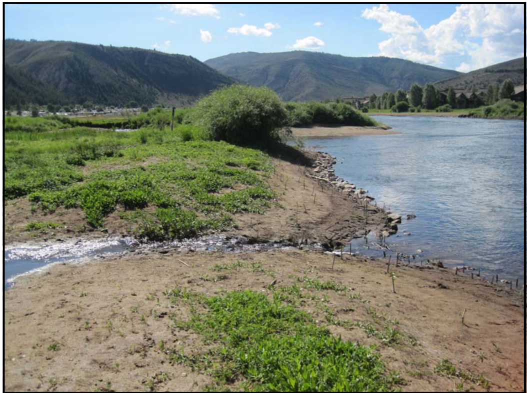
Point 2V1L: 8-15-11 Treatment area 2-10 after fence removal, bank layback, willow wattle installation, and cobble toe reinforcement.
