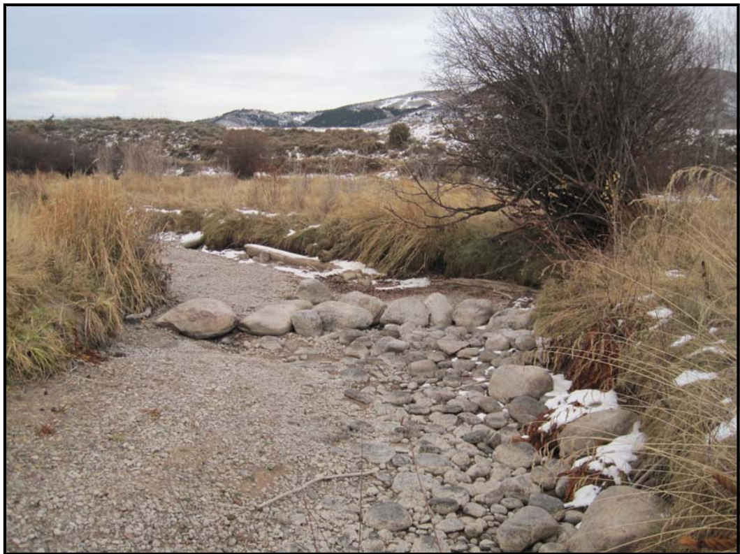
Point 1S6L: 11-11-11 Reach 5, left bank, looking upstream to existing grade control augmentation. Habitat logs are also visible.
