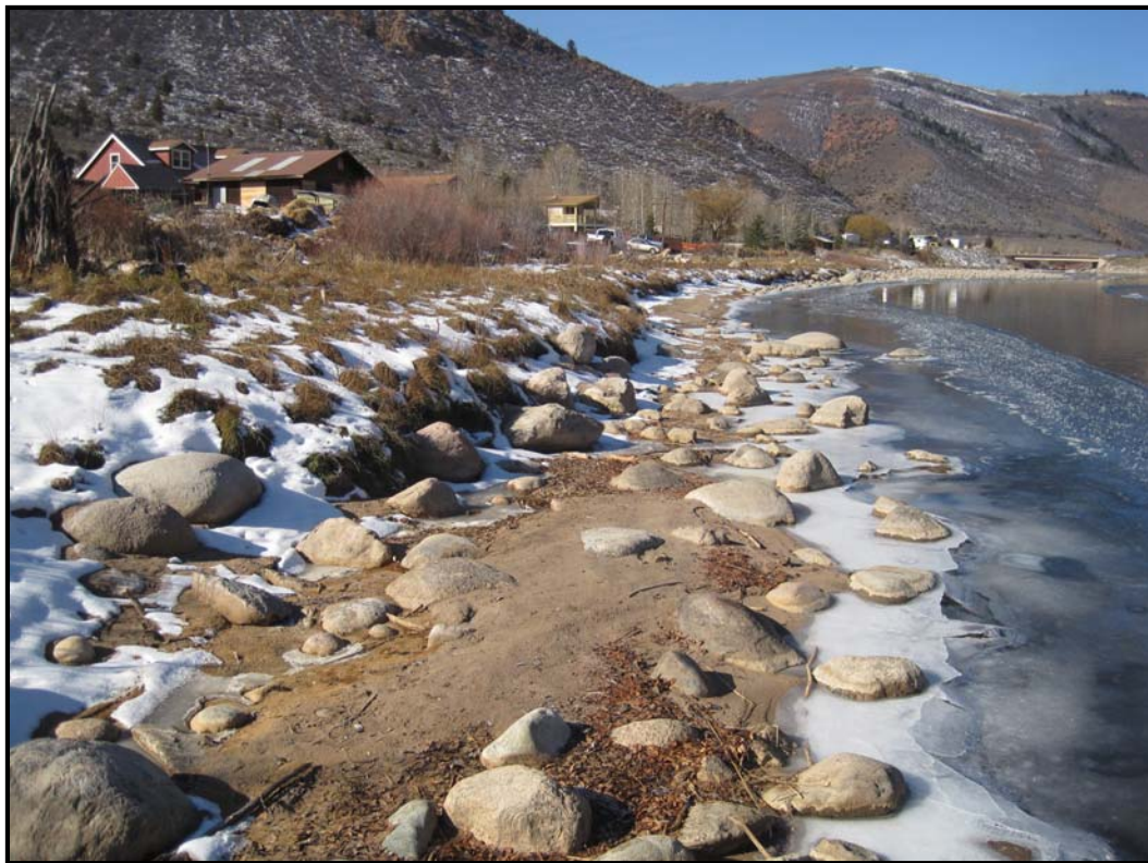
Point 1S3L: 11-11-11 Reach 2, looking downstream along Boulder/cobble Toe Treatment 1-16.
