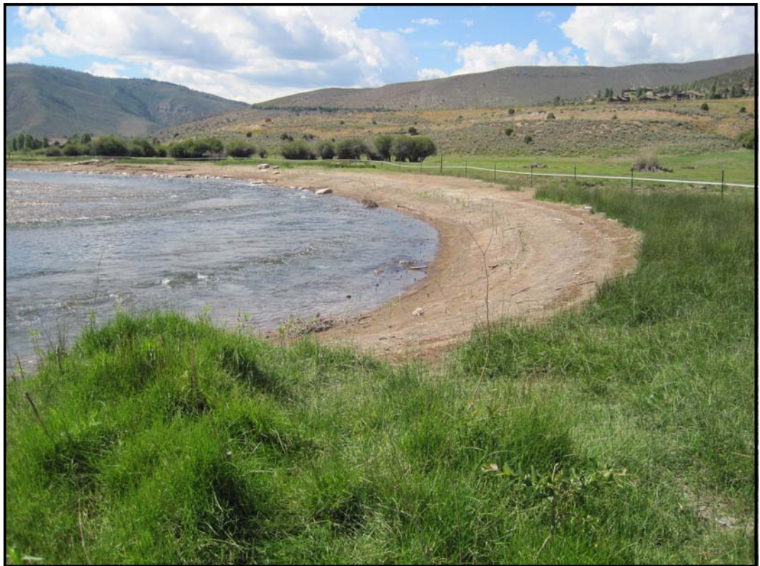
Point 2V4R: 8-15-101 Treatment area 2-6 after bank layback, willow wattle installation, and cobble toe reinforcement.
