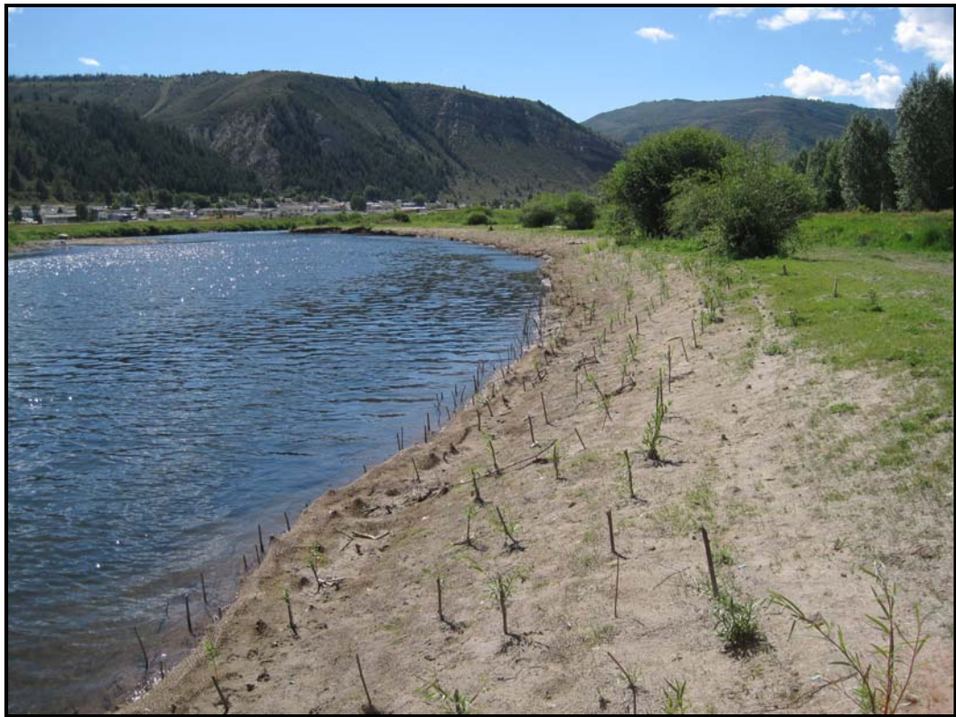
Point 2V1R: 8-15-11 Treatment area 2-13 looking downstream, 1 year after bank layback and willow wattle installation. (Willow wattles are underneath erosion control blanket at toe of slope.)
