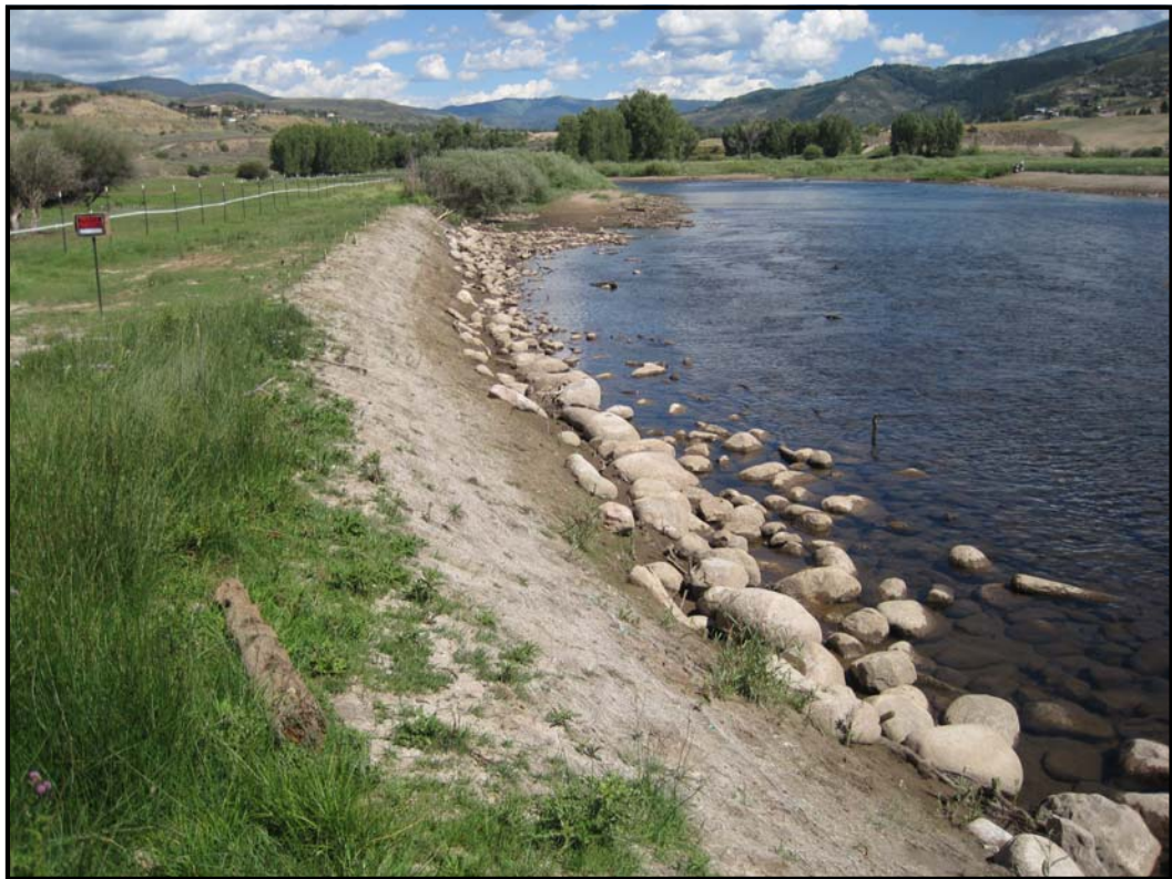
Point 2S1R: 8-15-11 Treatment area 2-11 after bank layback, willow wattle installation, and cobble bar enhancement. Fence was moved northward (to the left) to keep cattle off the river bank.
