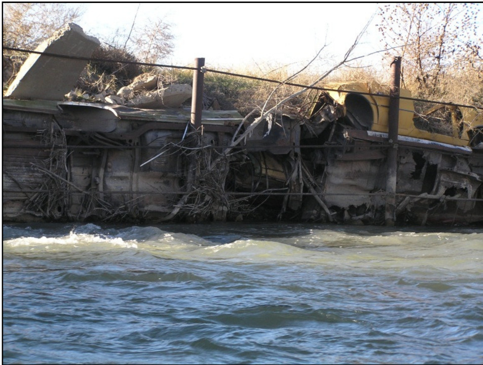
Figure 11: Picture of poorly engineered bank stabilization in the Animas River, NM.
