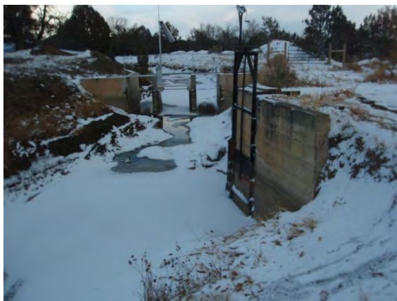
Hermana Ditch check structure and May Pipeline Slide Gate.
