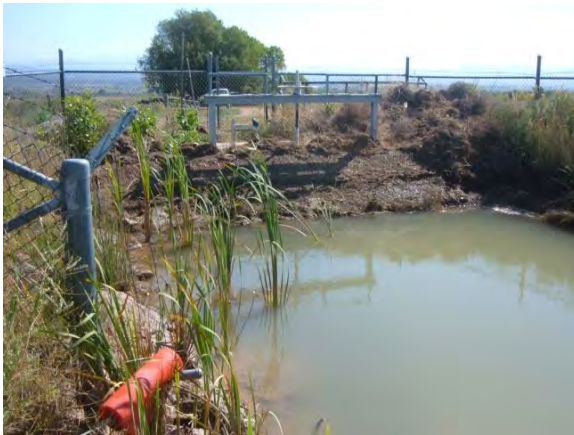
Lone Pine Pipeline Inlet existing screen covered with debris
