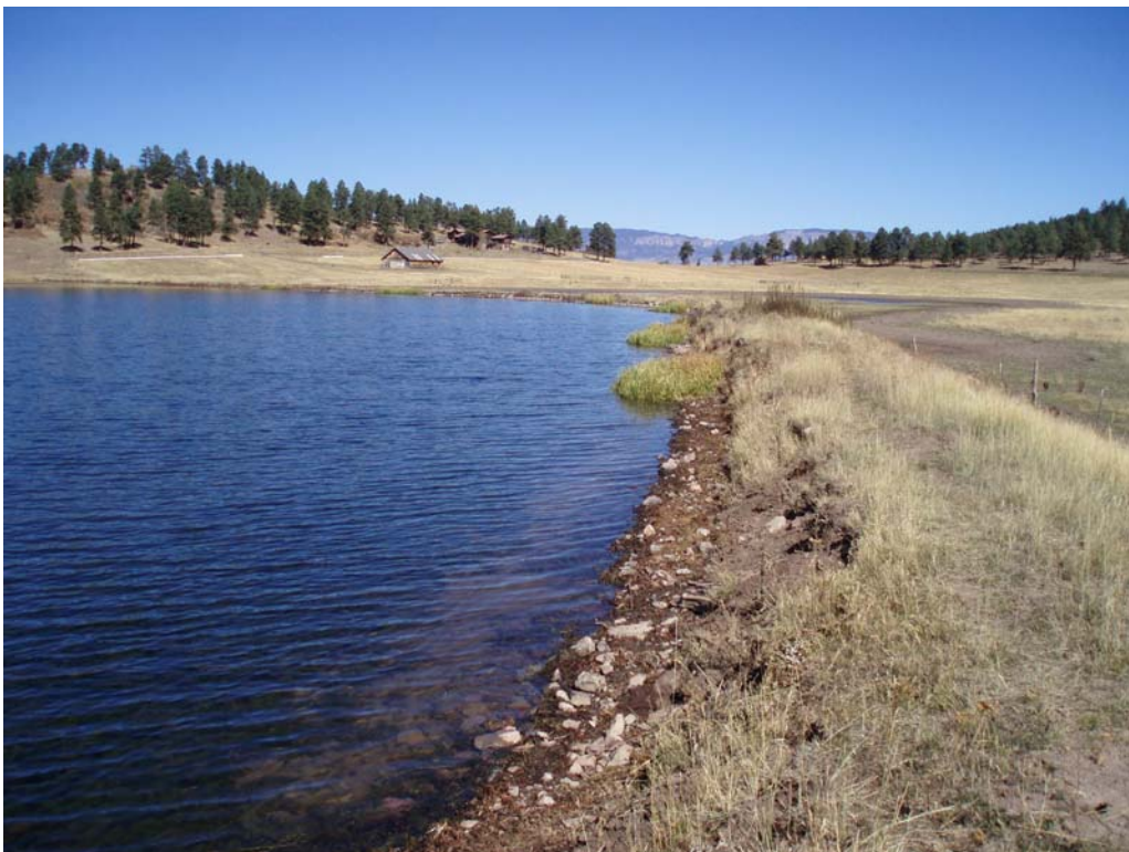
Typical shoreline along dike on east side of reservoir. Note wave action has eroded the dike and only patches of wetland fringe can persist here.
