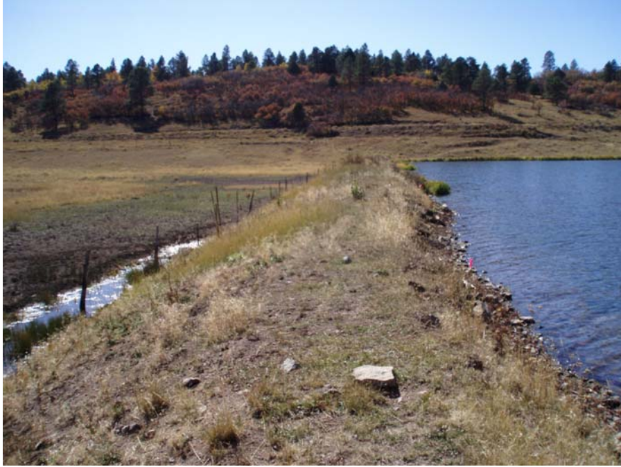
Existing dam/dike for the Reservoir. The intent was to contain water on Town property and not allow flooding onto adjacent private land. The dam is in need of repairs.
