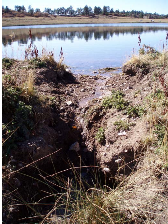
Photo of one of four breach locations along the existing dam. The breaches allow water to spill onto the adjacent property when the reservoir is full or during storms with wave action, extending the created wetland area beyond the Town property.
