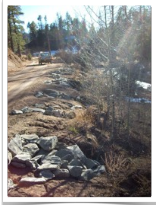
Before and after: erosion along side of Trail Creek Road, and rock placed to reduce continuing problem.
