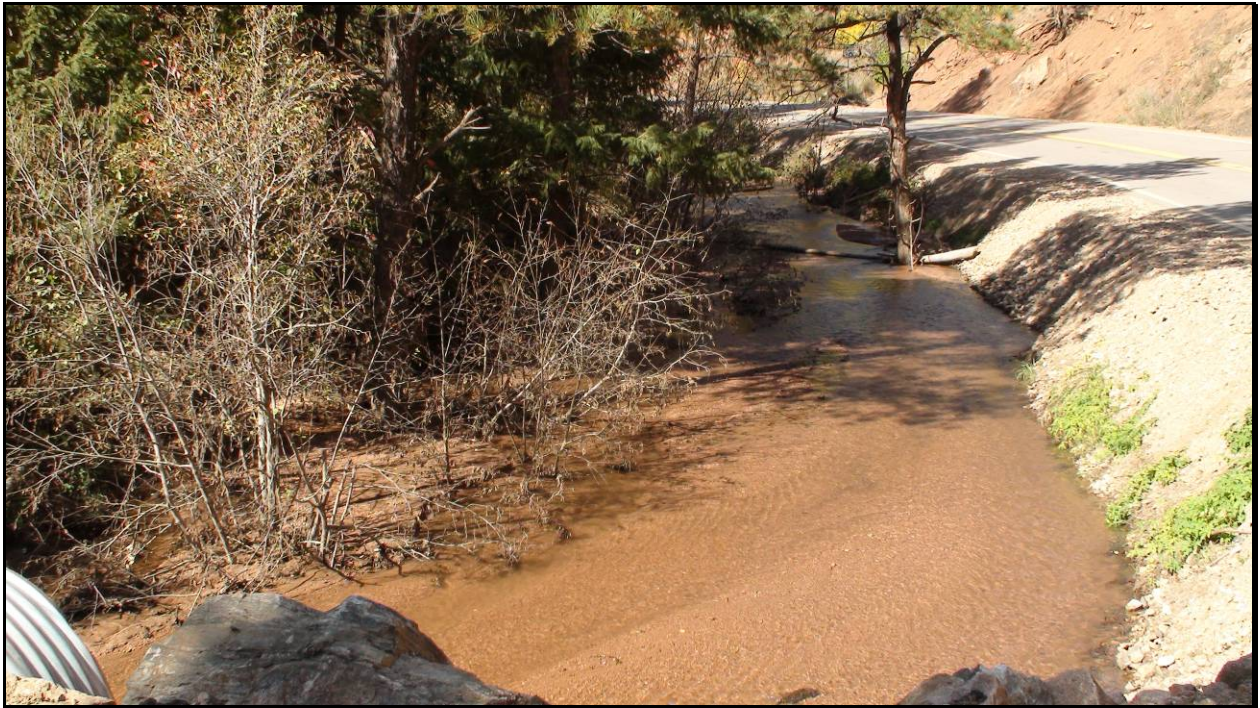
Figure 6. Road fill erosion due to channel encroachment, F4 stream type.
