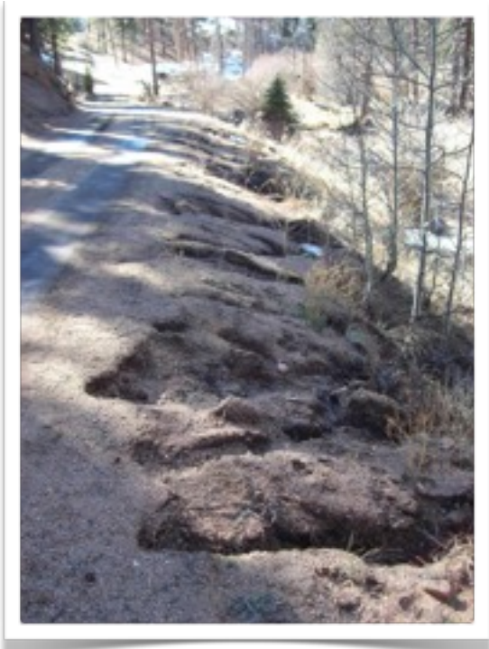
Before and after: erosion along side of Trail Creek Road, and rock placed to reduce continuing problem.
