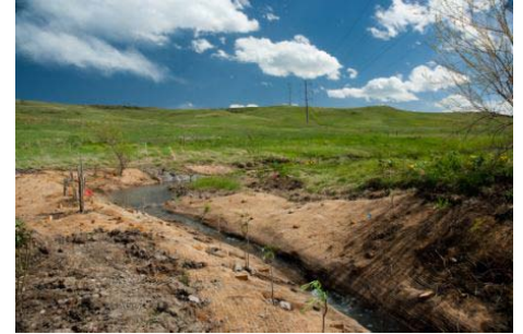
Re-graded Banks, Seeding, Erosion Matting, Planting, 2010
