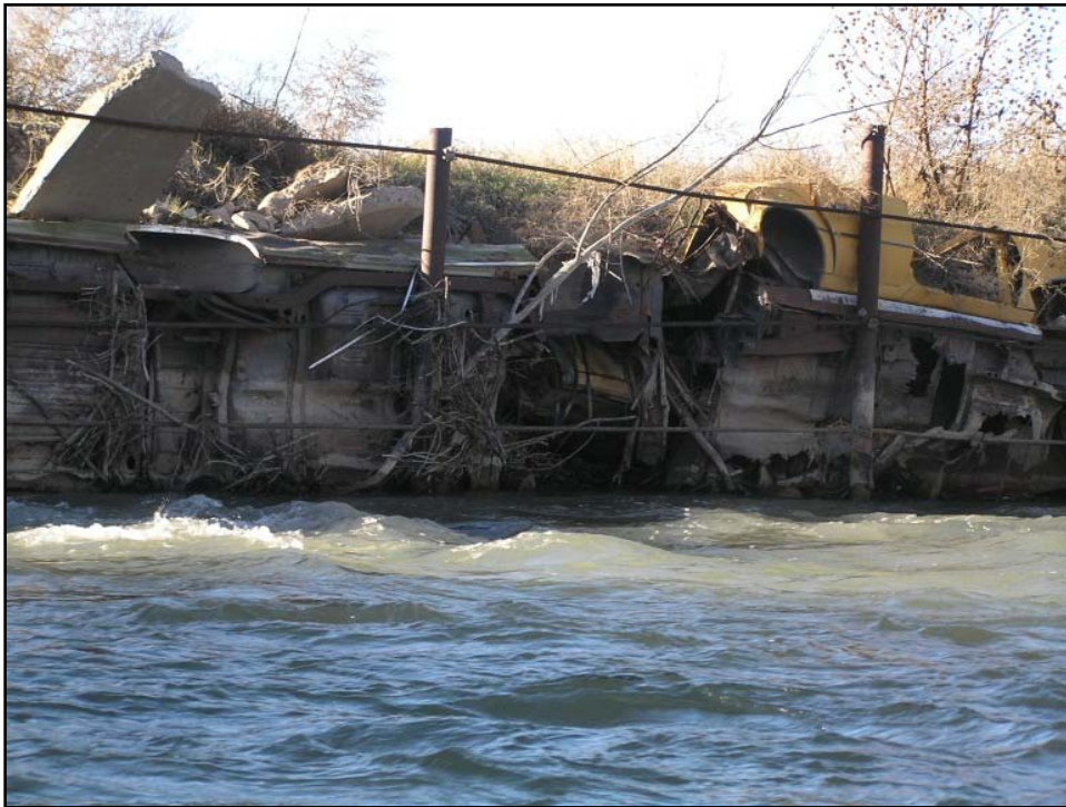
Figure 9: Picture of poorly engineered bank stabilization in the Animas River, NM.
