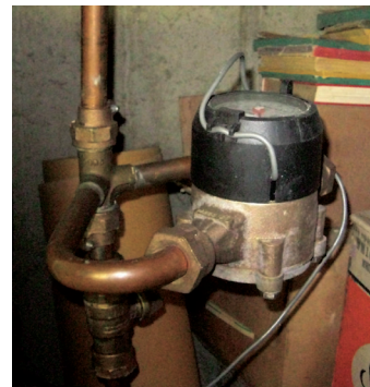
A new water meter is installed in a Brighton residence following the City's water audit program.
