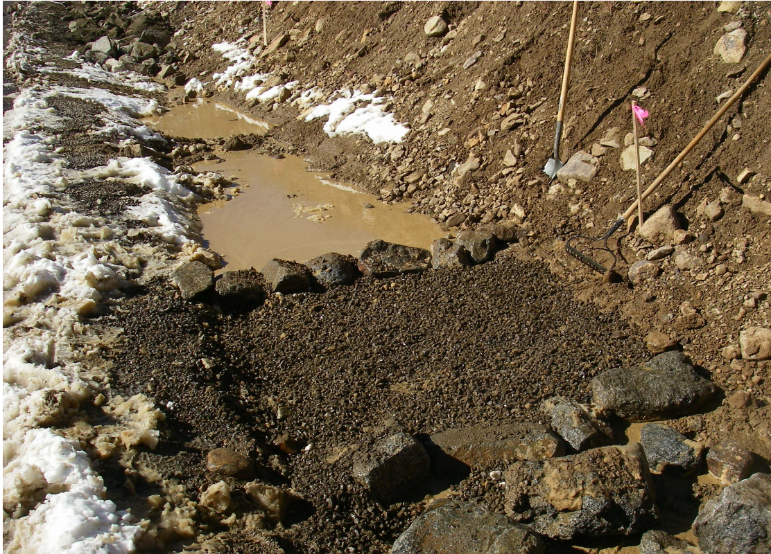
Figure 3- A rock check dam with an upstream stilling basin and downstream reinforced vegetative swale near Crested Butte, Colorado. A larger cap rock was installed to complete the check dam.
