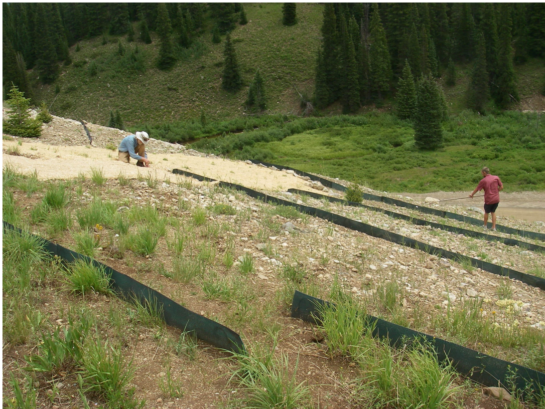
Figure 4 – Erosion control mats and “s-fence” being installed to address erosion on slopes in the Coal Creek Watershed, near Crested Butte, Colorado.
