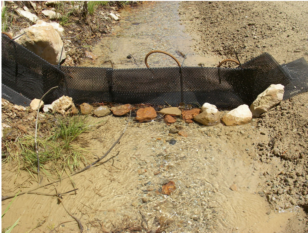
Figure 6 - "Ditch guard" check dams used to reduce roadside runoff on Kebler Pass Road near Crested Butte, Colorado.
