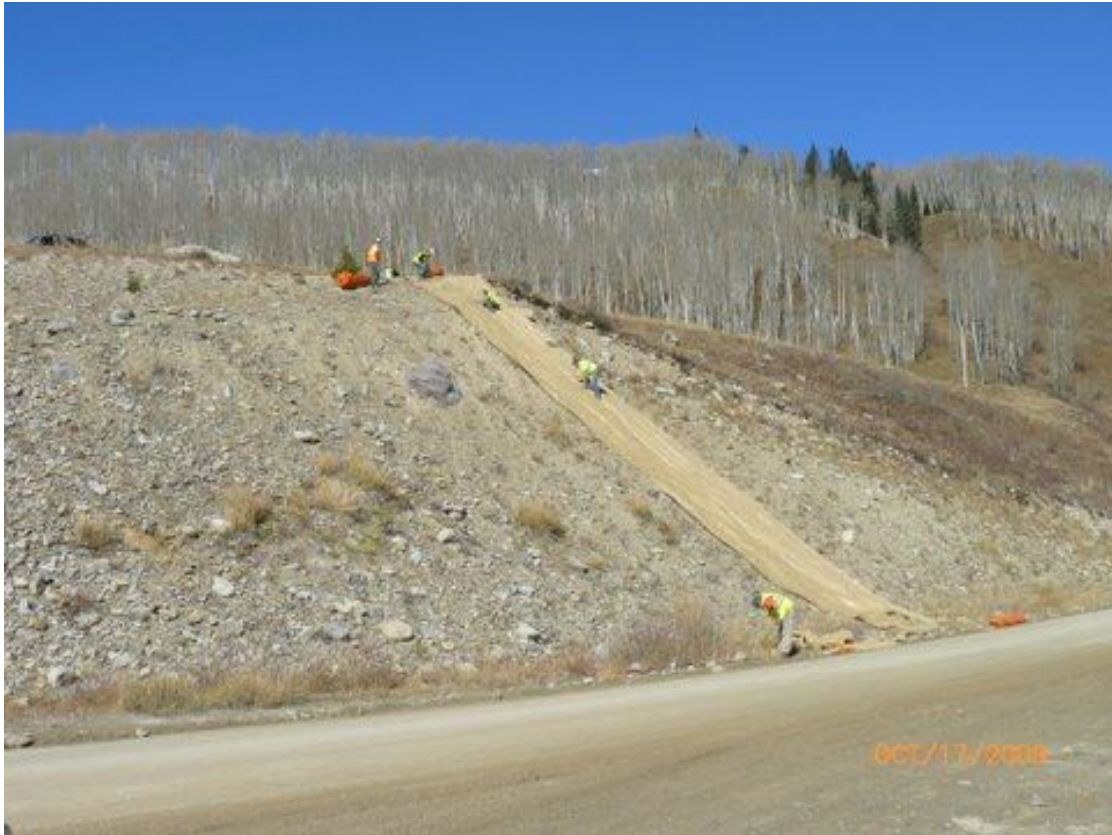
Figure 2 - Erosion control mats being installed in the Coal Creek Watershed near Crested Butte, Colorado, in 2009.
