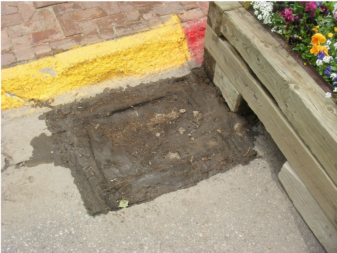
Figure 5 - "Grate guard" filters used to capture stormwater contaminants on Elk Ave in Crested Butte, Colorado.
