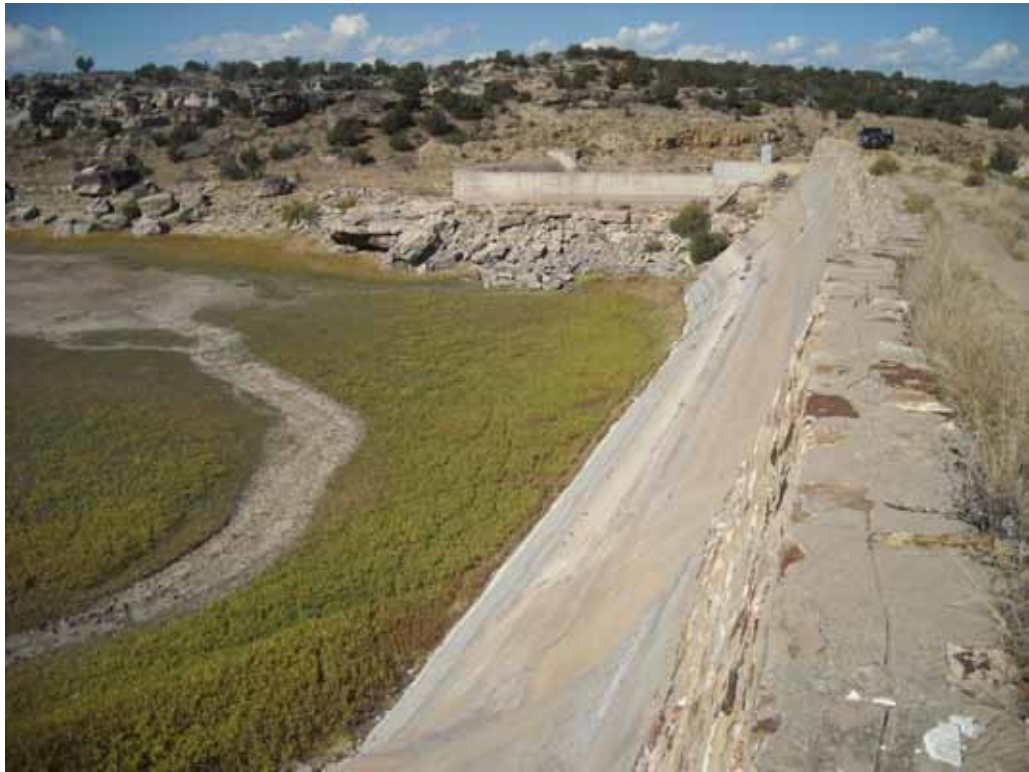
Photo 1. Cucharas Dam looking west along crest with ogee spillway in center background
