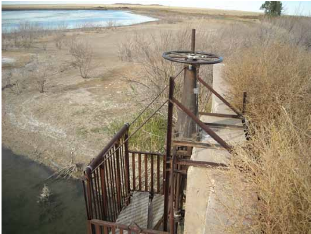
Photo 19. Huerfano Valley Reservoir outlet gate.
