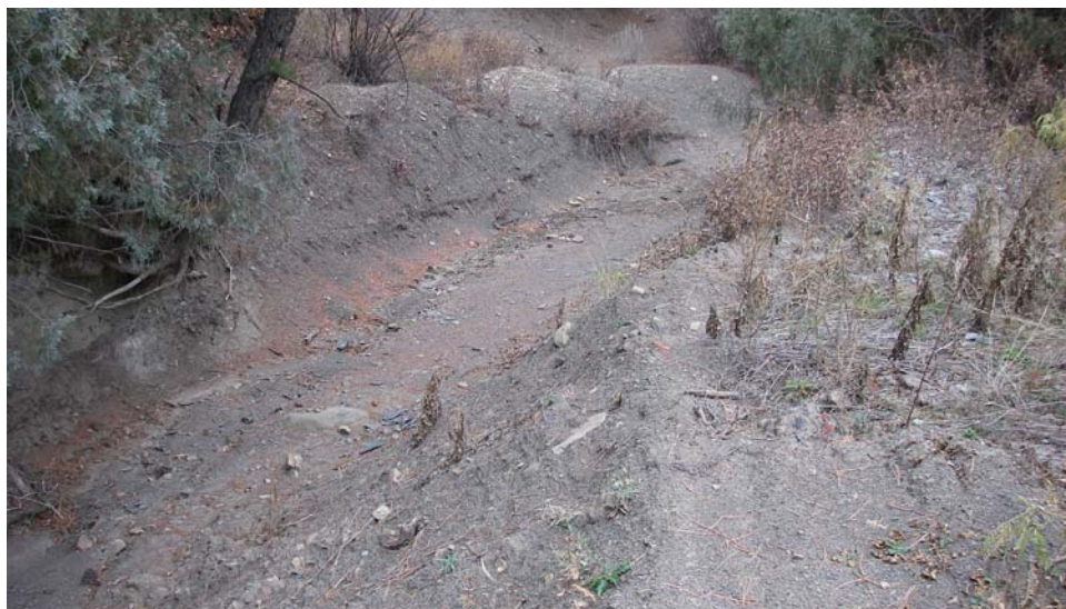
Photo 58. Upstream view showing highly incised channel due to excavation and berming activities (> 95% shale).
