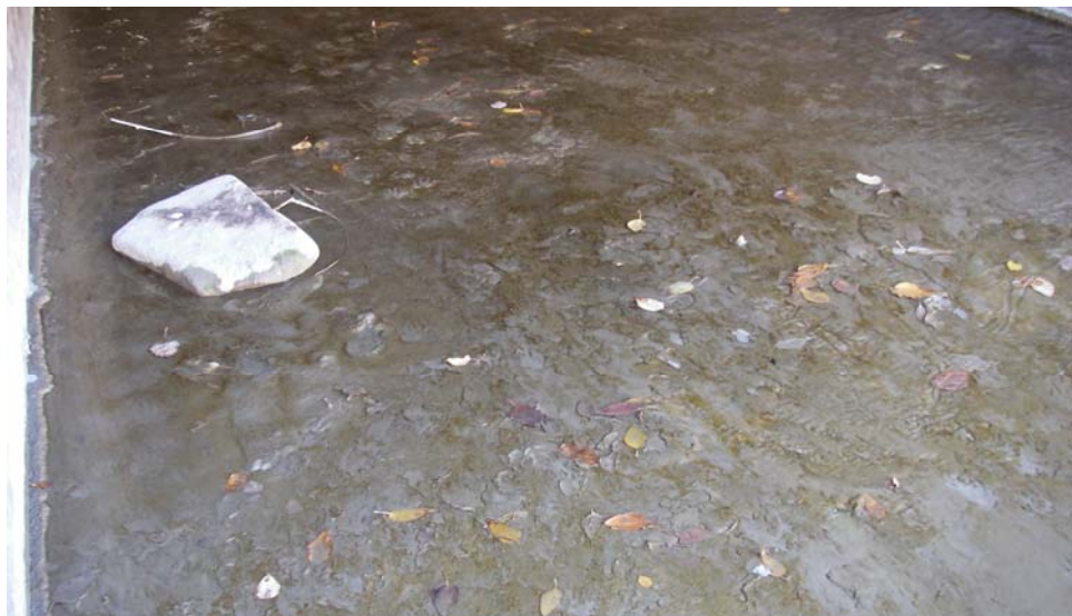
Photo 45. Upstream view of Wildcat Canyon/Hwy 160 culvert outlet (lots of fines with no shale material apparent).
