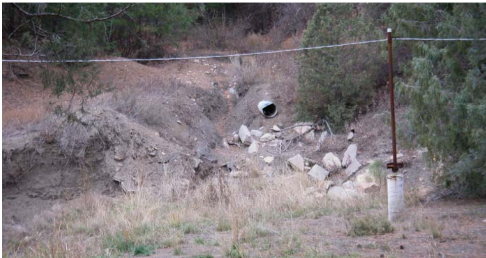
Photo 55. Point-source for erosion due to headcutting (probably due to drainage modifications).
