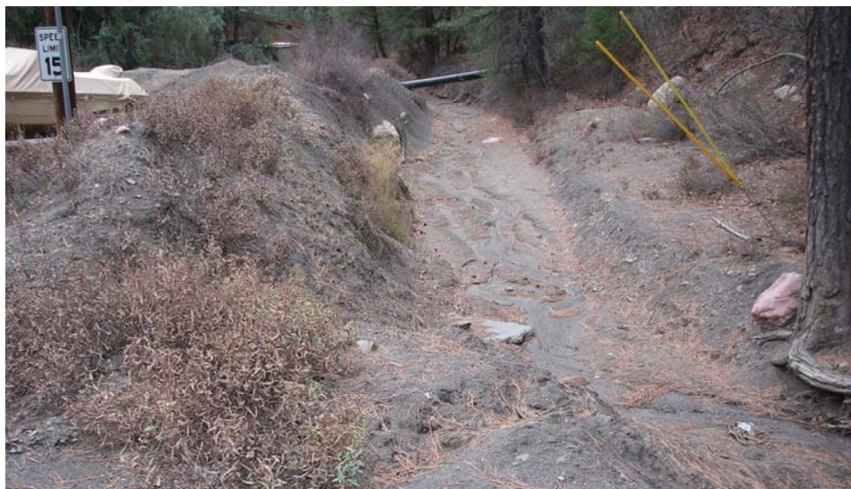
Photo 57. Downstream view showing highly incised channel due to excavation and berming activities (> 95% shale).
