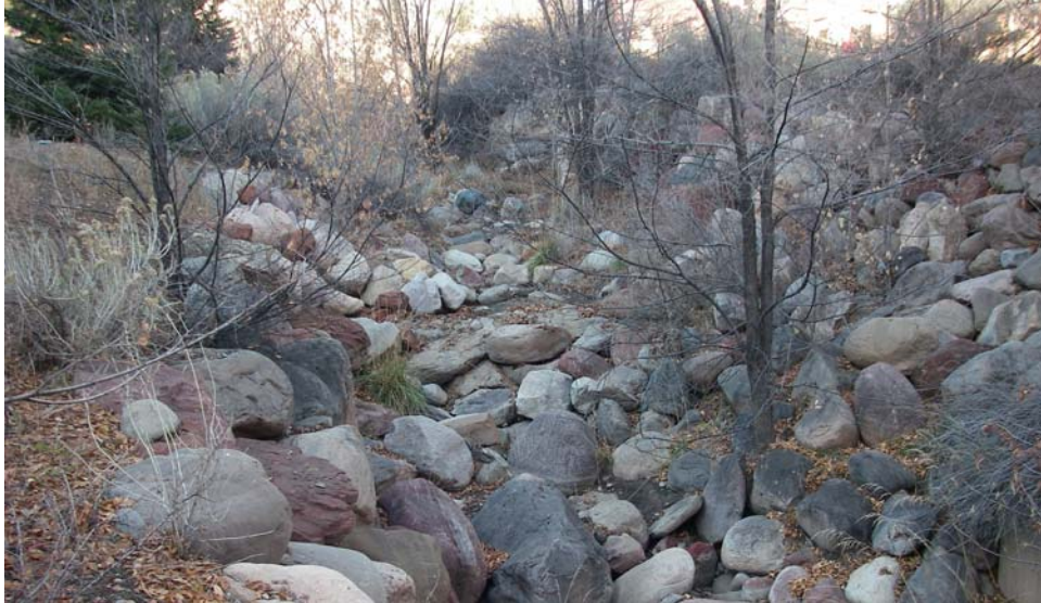
Photo 47. Upstream view of armored Tech Center channel along Tech Center Drive.
