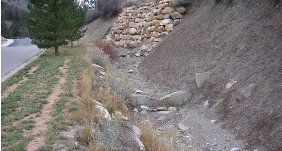
Photo 53. Upstream view of constructed channel with grade control structures ~ 300' upstream from Lightner Creek confluence (opposite Westwood Apartments).
