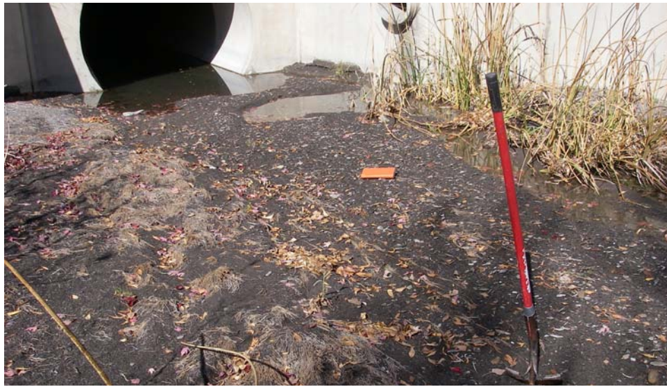
Photo 13. Depositional area at culvert outlet (predominately shale).
