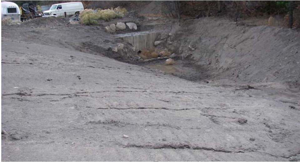
Photo 48. Downstream view of City sedimentation basin with low-elevation culvert outlet, high-elevation large capacity outlet and overflow spillway.
