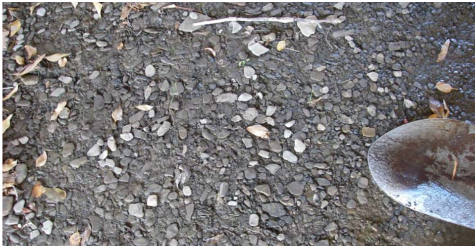
Photo 7. Depositional material (shale) in box culvert at Camper World entrance.
