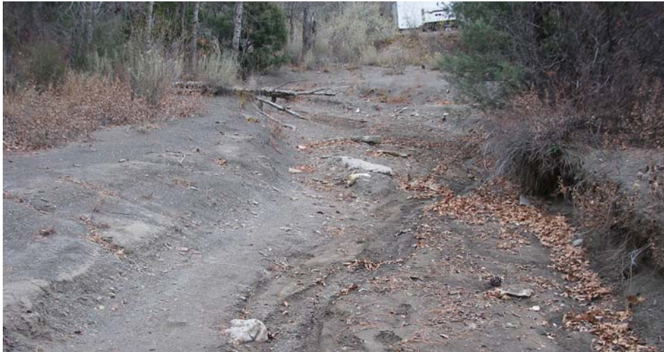
Photo 54. Upstream view of Perins Canyon channel at downstream end of single family residential area and at channel stability and sediment size analysis site. At least 95% shale composition.
