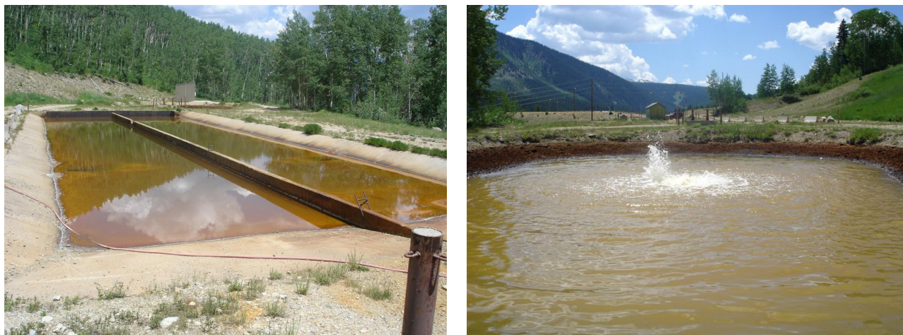
Figure 32. Photographs of the grit chamber (left) and equalization pond (right) used by the Mount Emmons treatment plant. The chamber and pond are located above the Keystone Mine drainage that forms part of unnamed tributary UT-5.368.
