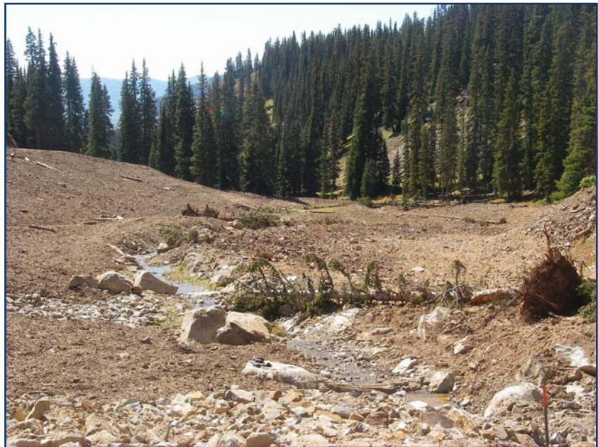
Figure 7. A view of the new Elk Creek with fallen trees, rock features, and vegetation incorporated into the design to mimic a natural creek.
